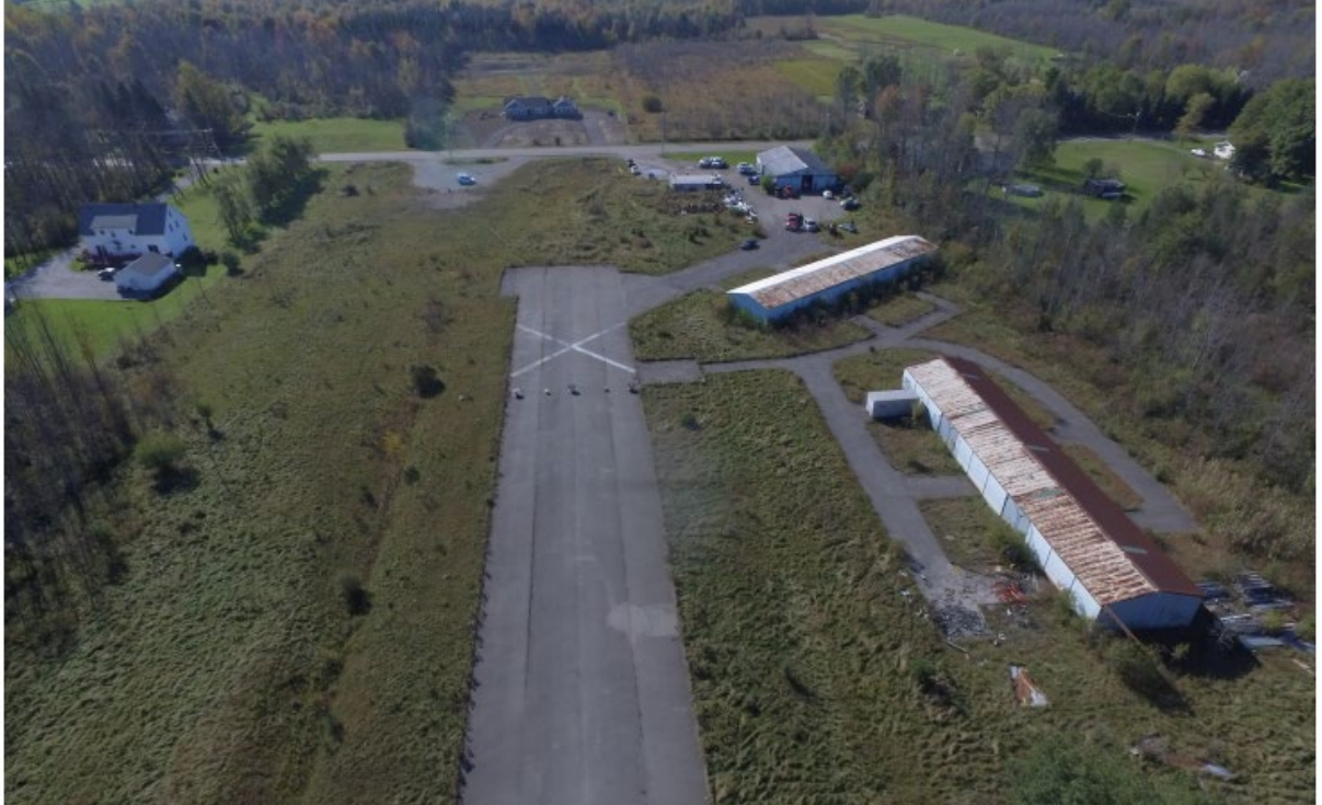
Former runway to be connected to Eden Evans Center Road to form new industrial road, buildings to be demolished.
