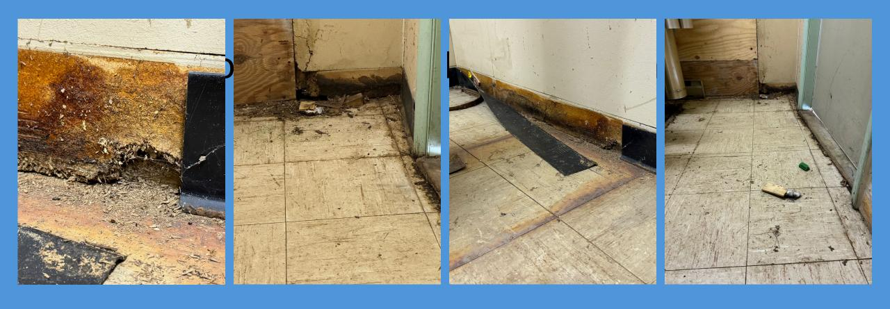
Walls & Footers deteriorated due to past water damage and mice
