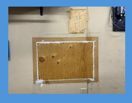
Walls patched where old fans & air conditioners were removed (note water leak)
