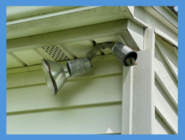
• Flood light fixtures on front and rear corners of shelter not adequate to provide secure environment at night
