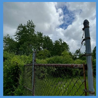
Gate does not secure properly and barbed wire has rusted, deteriorated and is no longer viable
