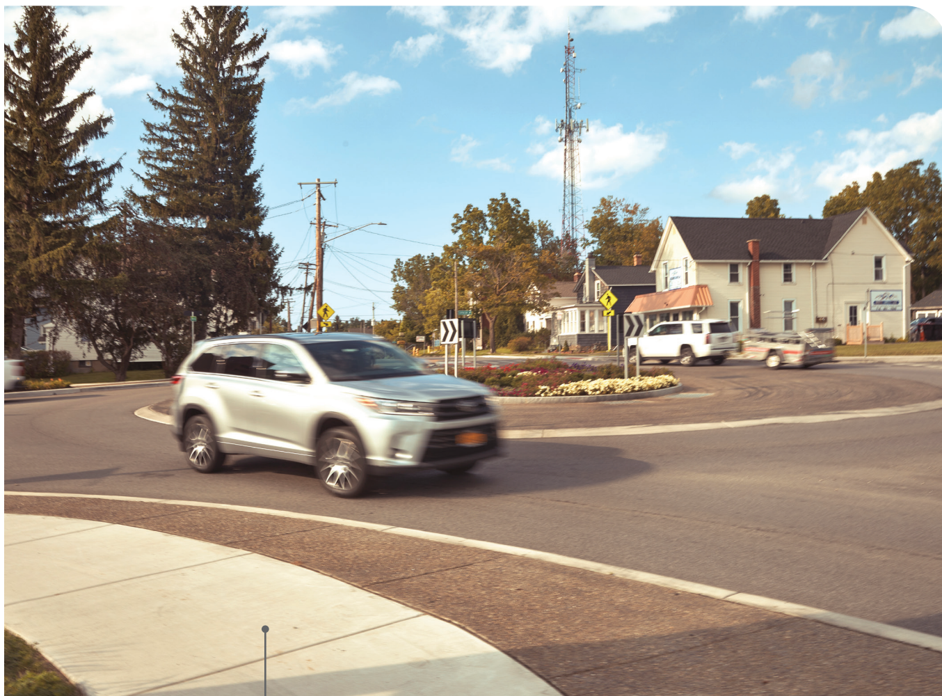
Traffic signals were replaced with two landscaped roundabouts in the Village of Lancaster as part of its West Main Street Extension Project. The slower but safer and more efficient flow of traffic has led to a reduction in emissions and intersection delays.
