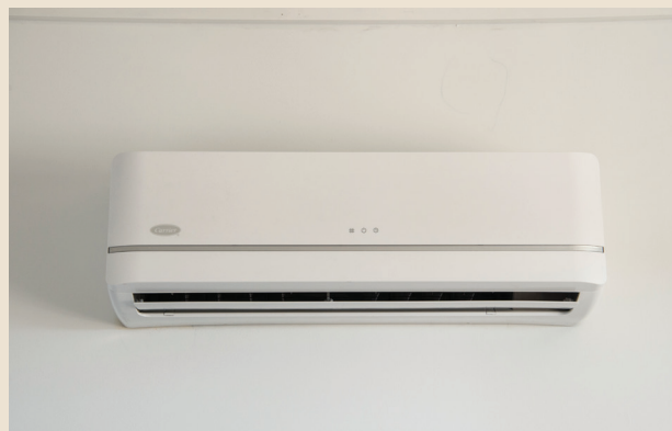
Ductless air source heat pump indoor unit.
