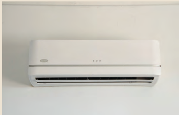
Ductless air source heat pump indoor unit.
