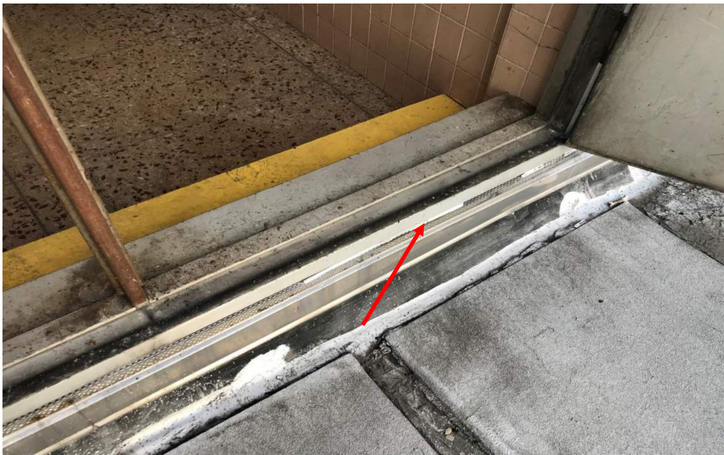
Photo 1: Photograph of white door caulk associated with the West Penthouse doors. The caulk was determined to be PCB-containing.
