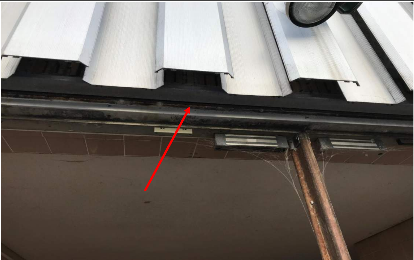
Photo 1: Photograph of white door caulk associated with the West Penthouse doors. The caulk was determined to be PCB-containing.
