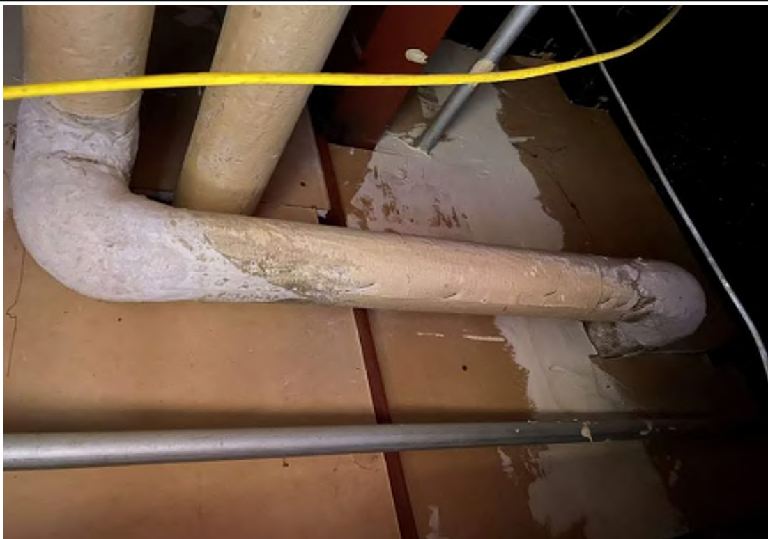
Photo #14 - View of mudded fittings on fiberglass pipe insulation above the suspended ceiling in Office 109, by the door to the corridor. Photo Date: 08/17/2023 The mudded fittings, paper jacket and tar in the jackets on fiberglass were determined to be non-asbestos.
