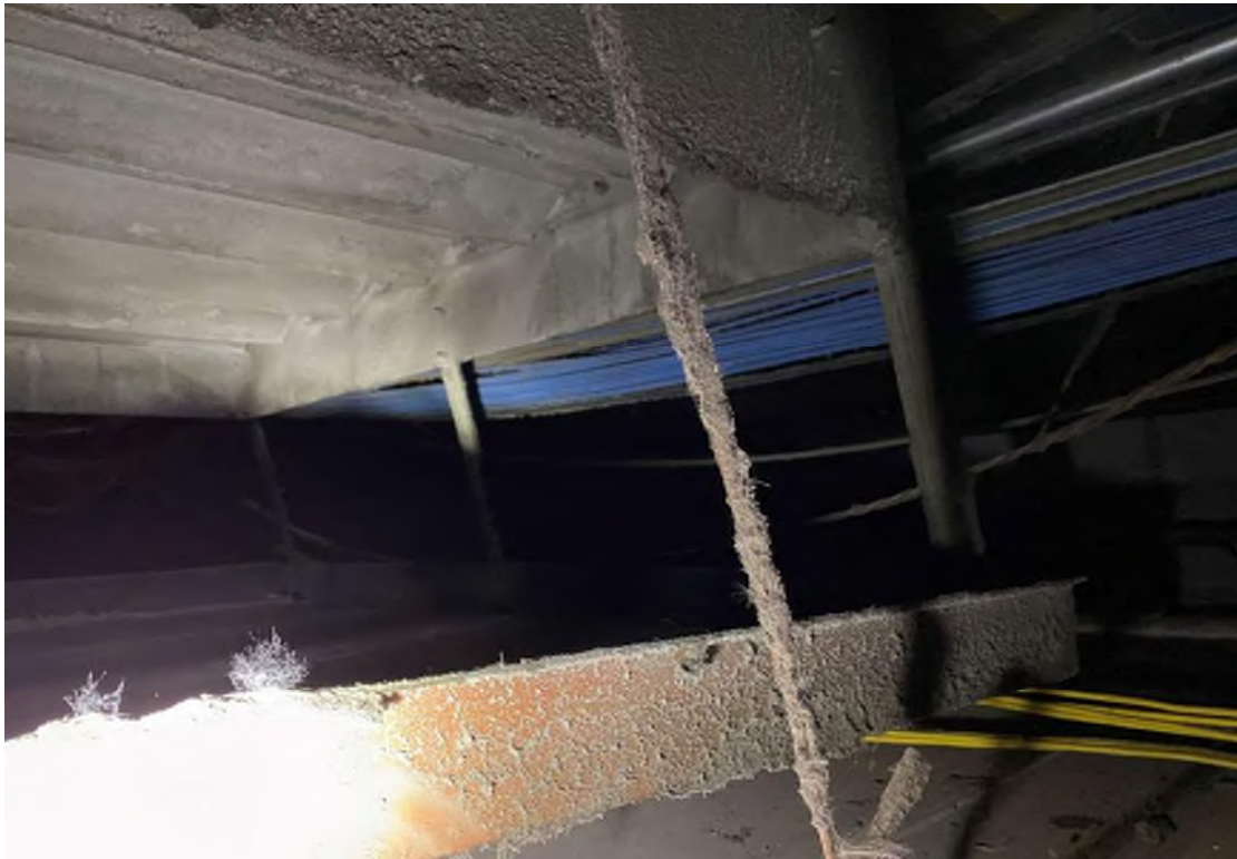
Photo #12 - View of large HVAC duct and the base of a roof top AHU above second floor corridor suspended ceiling tiles by Classroom 234. Photo Date: 08/18/2023 No insulation or suspect asbestos-containing stickpin mastic was observed on accessible corridor ducts.
