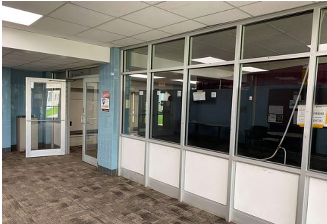
Photo #8 - View of the windows in Lobby 168 abutting Student Lounge 123 in the center area of the first floor corridor. The window frame caulk was determined to be non-ACM and non-PCB containing. Window glazing compound was determined to be non-ACM. Carpet adhesive on terrazzo and ceiling tiles were determined to be non-ACM. Photo Date: 08/17/2023
