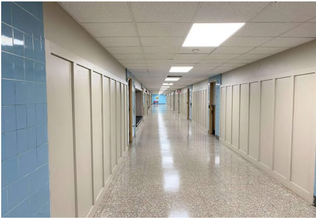
Photo #3 - View of plywood paneling and the corridor upper plaster walls on the second floor where lockers have been removed. Wall plaster in the building has been determined to be non-ACM. Blue ceramic wall tiles abutting doorways to classrooms has been determined to be an asbestos-containing material. Metal ash urns are set in blue ceramic wall tiles. Photo Date: 08/17/2023
