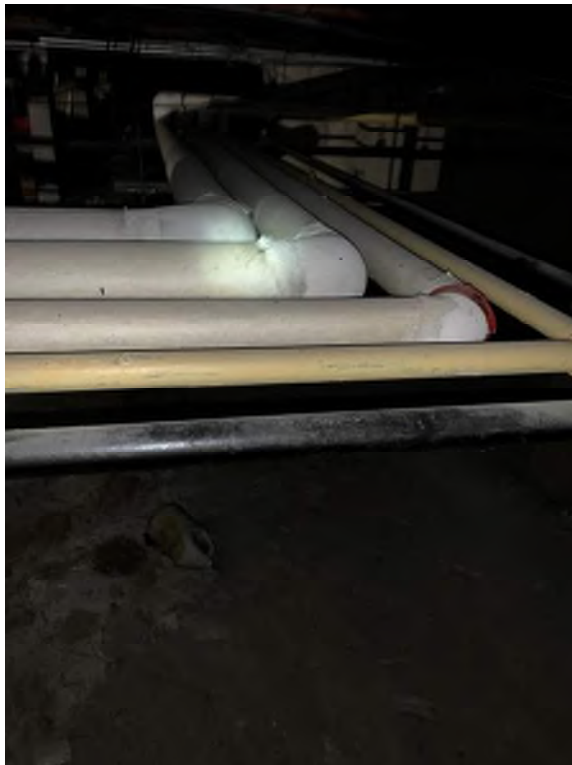
Photo #2: HAN 421- Kittinger Hall-Mud Fitting on Fiberglass Insulation
