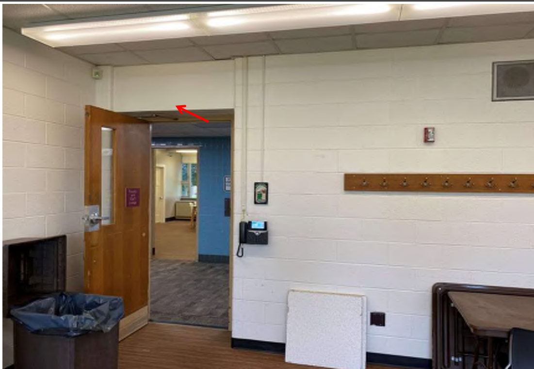
Photo #5 - View in Office 125 facing the corridor. The Paint on concrete masonry block walls was determined to be non-lead based paint. No caulk or sealant was observed along the steel door frames. Window glazing compound for the inset windows in the wood doors was determined to be an asbestos-containing material. Plaster above the door was determined to be non-ACM (arrow). Photo Date: 08/17/2023
