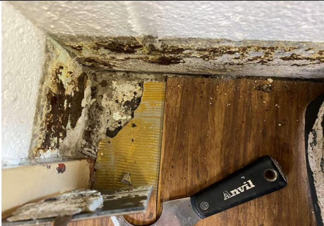
Photo #6 - View of non-ACM wood laminate-style sheet flooring on top of 9" asbestos-containing floor tiles in Room 125 by the door. Photo Date: 08/17/2023 All classrooms and offices in project limits have Asbestos-containing floor tiles beneath sheet flooring.
