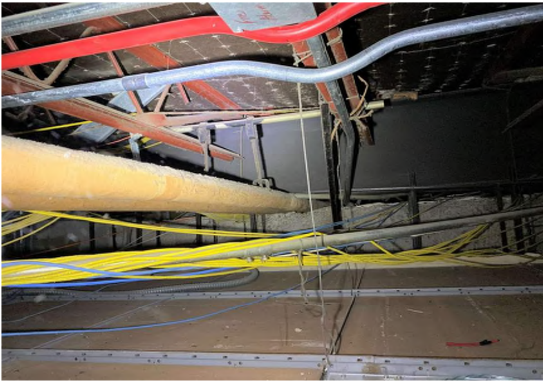
Photo #9 - View of fiberglass insulated piping above the suspended ceiling in Lobby 168. The paper with underlying black tar dabs on Photo Date: 08/17/2023 the fiberglass insulation was determined to be non-ACM. No mudded fittings were observed in this area.
