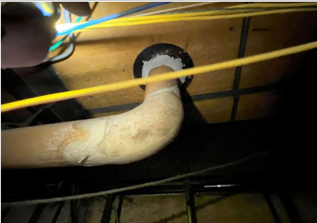
Photo #15 - View of a mudded insulation roof drain at the ceiling in the second floor corridor in front of Classroom 224.
