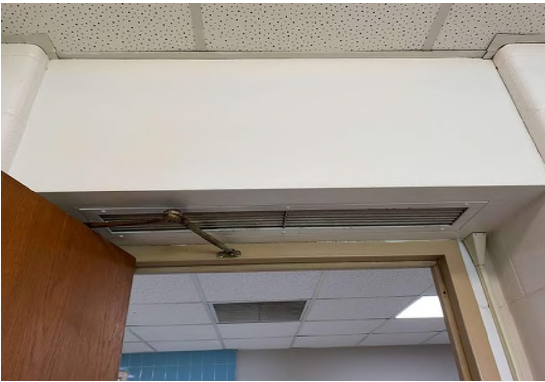
Photo #11 - View of the HVAC duct vent above the doorway in Classroom 234. No caulk or sealant was observed on the vent. Photo Date: 08/17/2023 The plaster was determined to be non-ACM. The ceiling tiles were also determined to be non-ACM.
