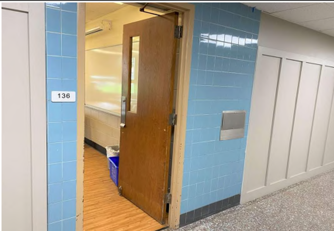
Photo #1 - View of the first floor corridor at Classroom 136. The thin set mastic associated with the blue ceramic wall tiles on the corridor walls has been determined to be an asbestos-containing material. Non-ACM terrazzo flooring is present in the corridors. Photo Date: 08/17/2023 Corridor and classroom suspended ceiling tiles have been determined to be non-ACM.
