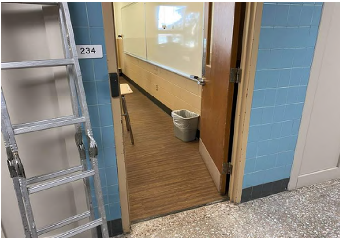
Photo #7 - View of the non-ACM sheet flooring on top of gray 9" asbestos-containing floor tiles in Classroom 234. Photo Date: 08/17/2023 Trace asbestos less than 1% was detected in the mastic behind vinyl cove base.
