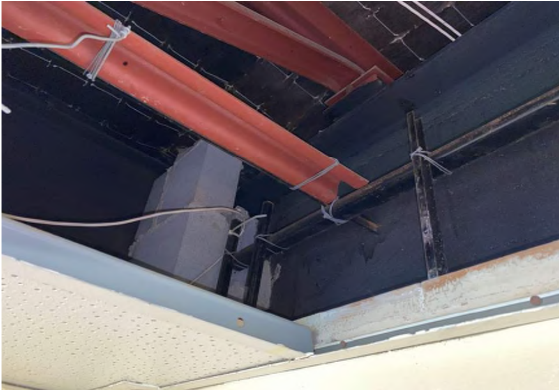
Photo #10 - View of the black structural steel beam above the HVAC vent in classroom 136. The black paint on the steel beams Photo Date: 08/17/2023 at the edges of corridor walls and above HVAC vents was determined to be lead-based paint.
