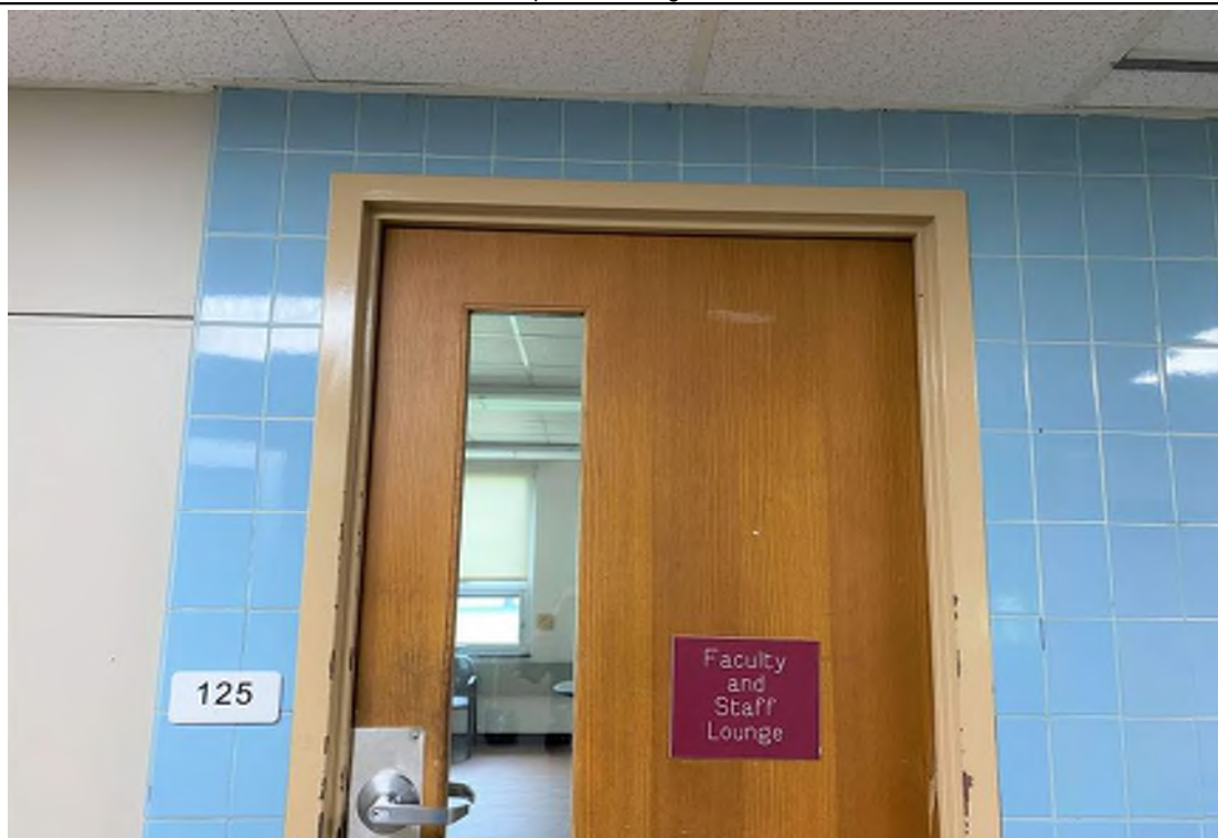
Photo #2 - View of the corridor wall and door to Room 125. The window glazing compound for the inset windows for the wood doors to classrooms and offices has been determined to be an asbestos-containing material. Photo Date: 08/17/2023
