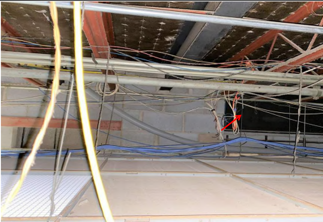
Photo #13 - View above the first floor corridor suspended ceiling tiles by Classroom 136. No spray-on fireproofing was observed on first floor or second floor decks above the suspended ceiling tiles. Paint on red girders was determined to be non-lead based paint. A steel beam with black lead-based paint above a doorway is visible in the concrete masonry block wall (Arrow). Photo Date: 08/17/2023
