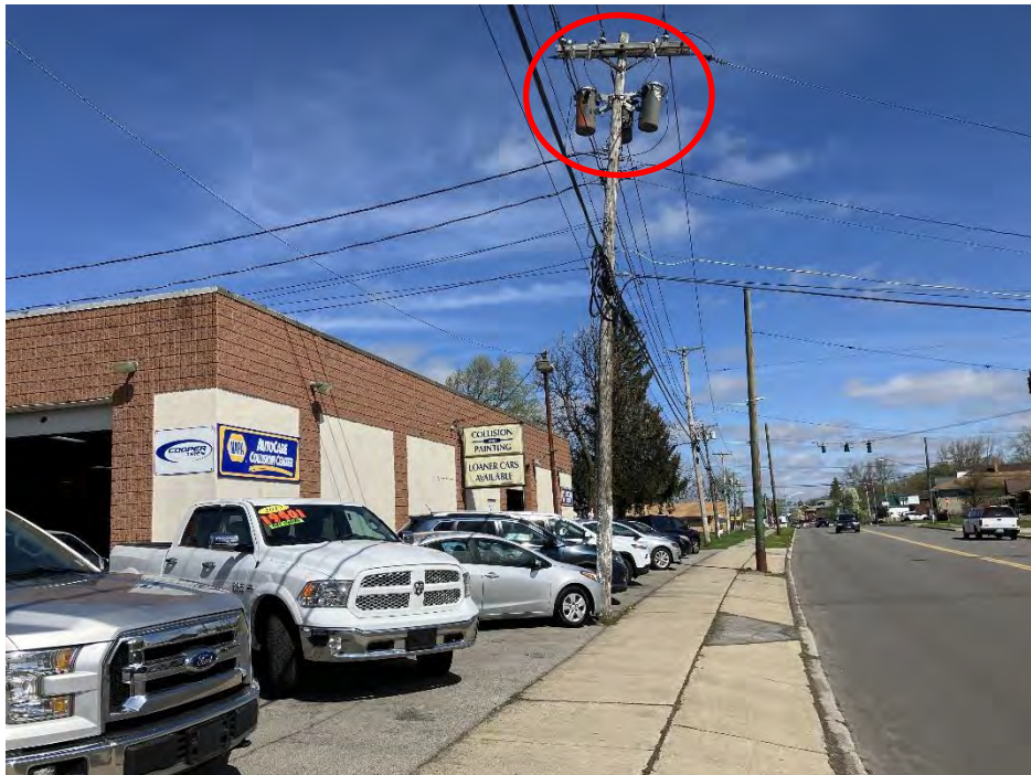
Photo 10 – Pole-mounted transformers throughout project corridor. Multiple transformers throughout the corridor are rusting. Unknown if any of the transformers contain PCB oil.
