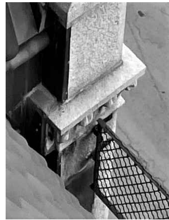
PHOTO #7: TYPICAL SMALL DORMER SNOW FENCE & BRACKET
