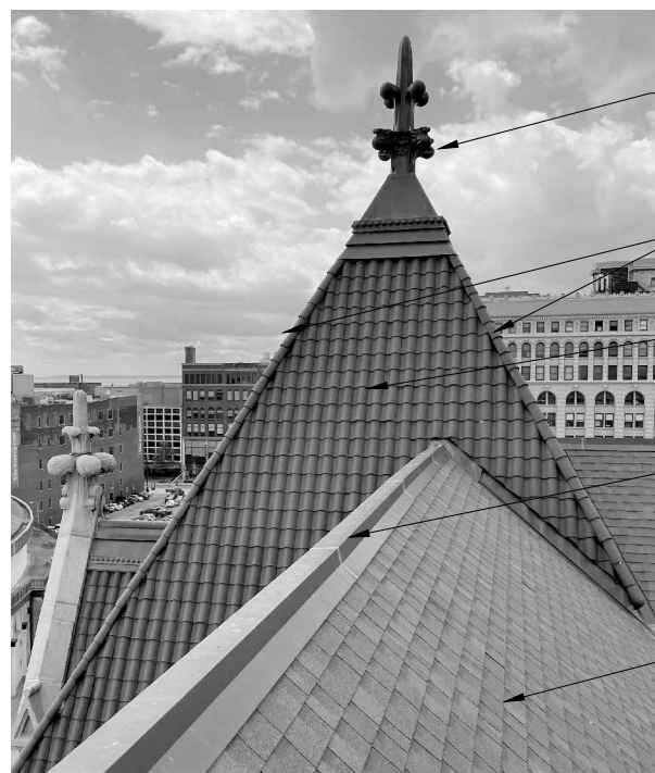
PHOTO #3: CORNER TURRET ROOF WITH COPPER FINIAL
