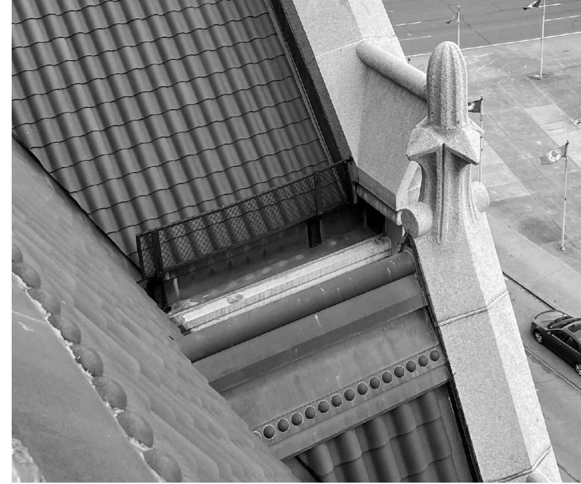
PHOTO #8: LARGE DORMER SNOW FENCE & BRACKET
