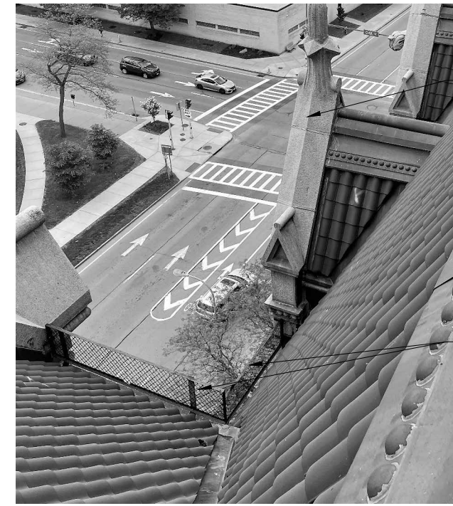
PHOTO #5: TYPICAL SMALL DORMER AND FRONT VALLEY
