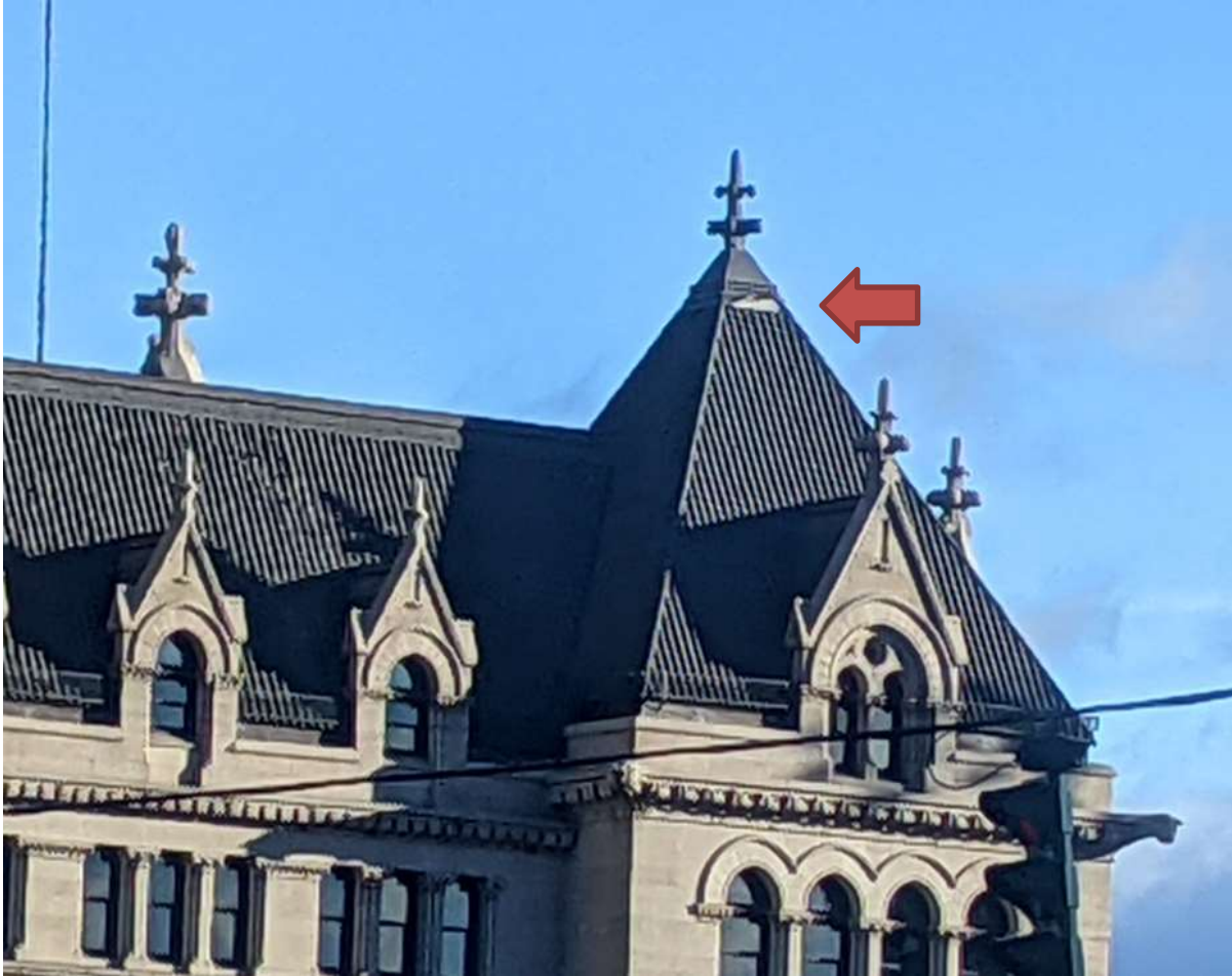
Southwest Copper Finial Skirt Damage on Roof 'R'
