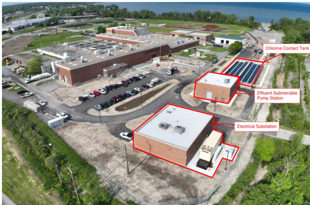
Figure 3. Phase 1 Built Improvements
