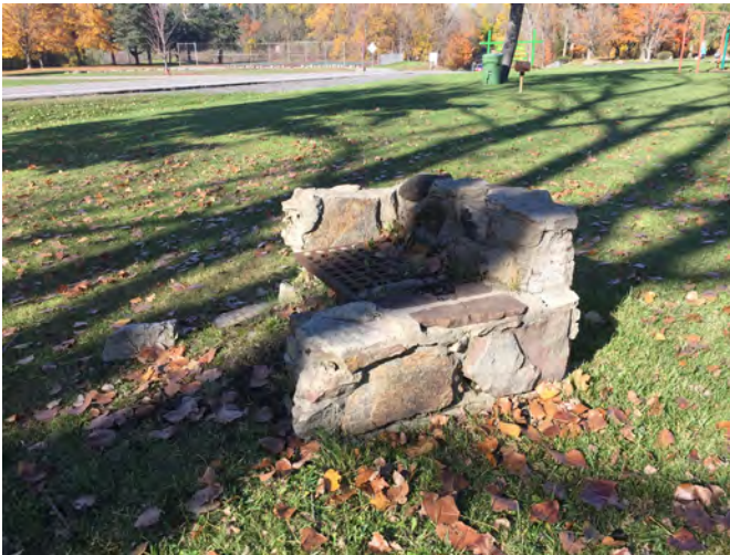
Old stone grill near Parkview Drive - All grills are displaying signs of deterioration like this throughout the park
