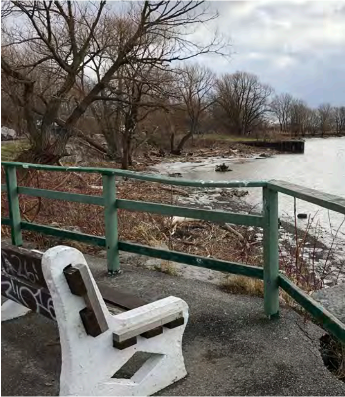
Railings in poor shape at the overlook area
