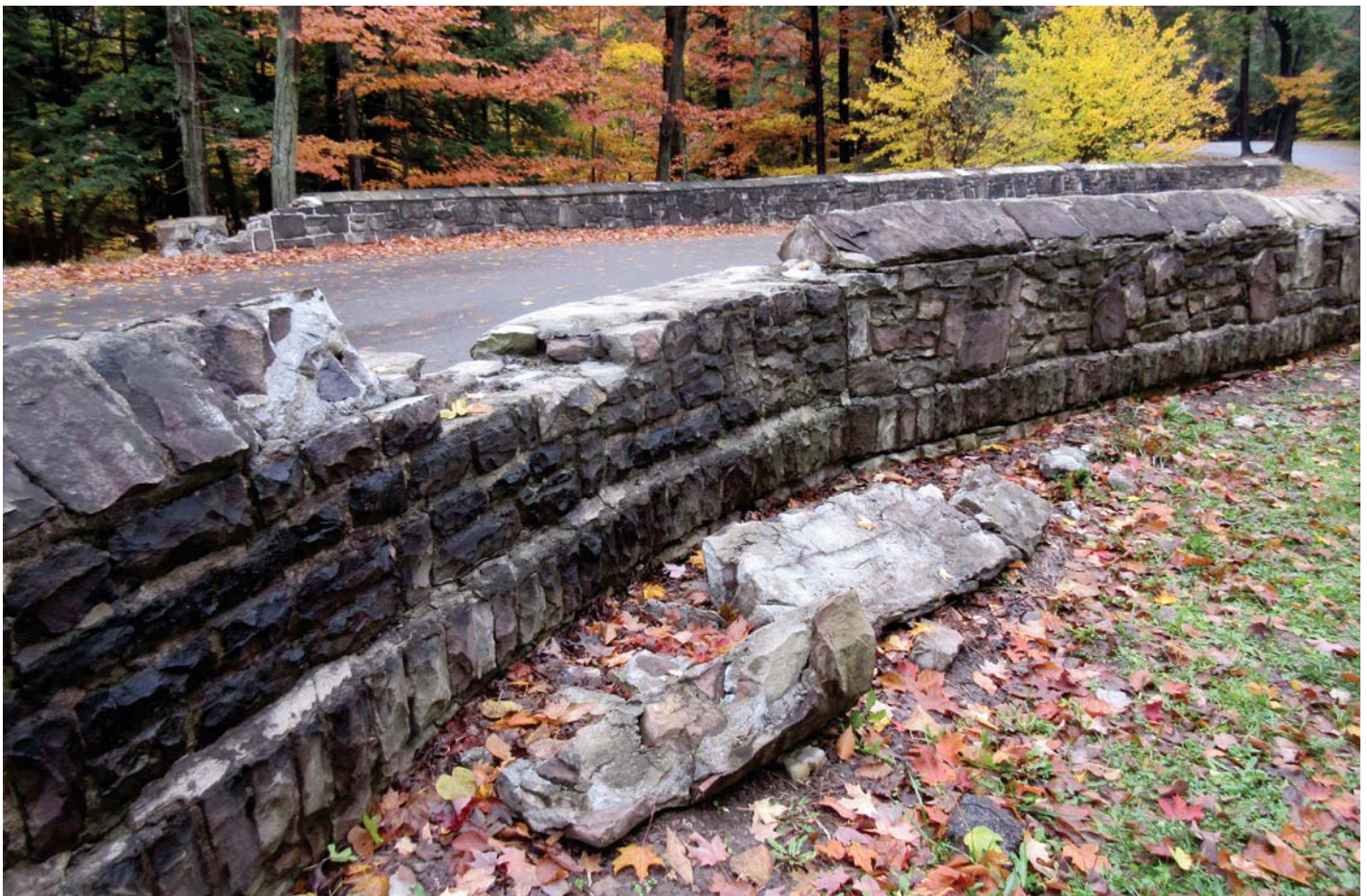
Stone work in need of repairs on WPA bridge at Chestnut Ridge Park
