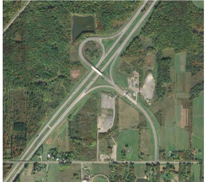
The existing Thruway interchange in Evans.
