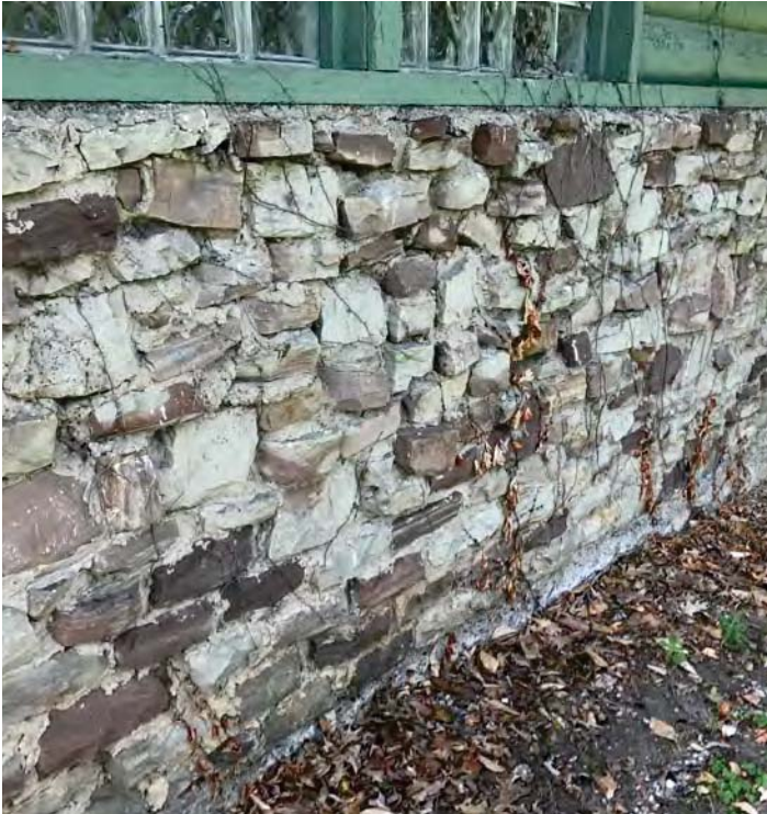
Stonework is starting to break apart at many shelters and structures
