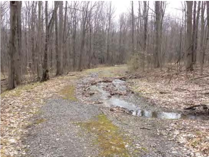
Drainage issues on the northern ravine trail
