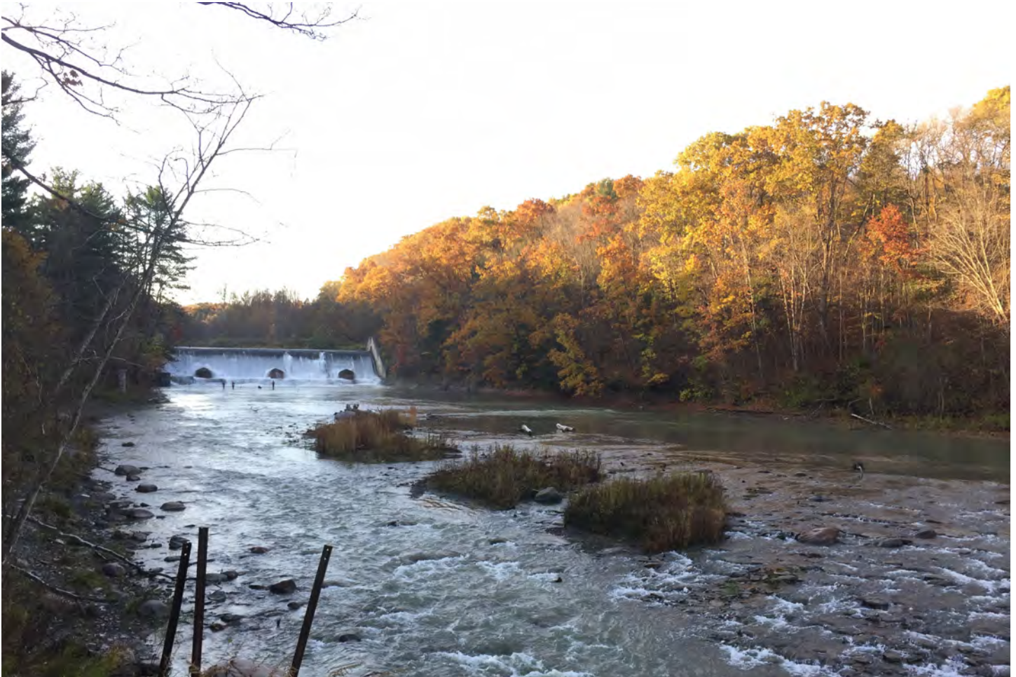
A view down Cattaraugus Creek towards the dam
