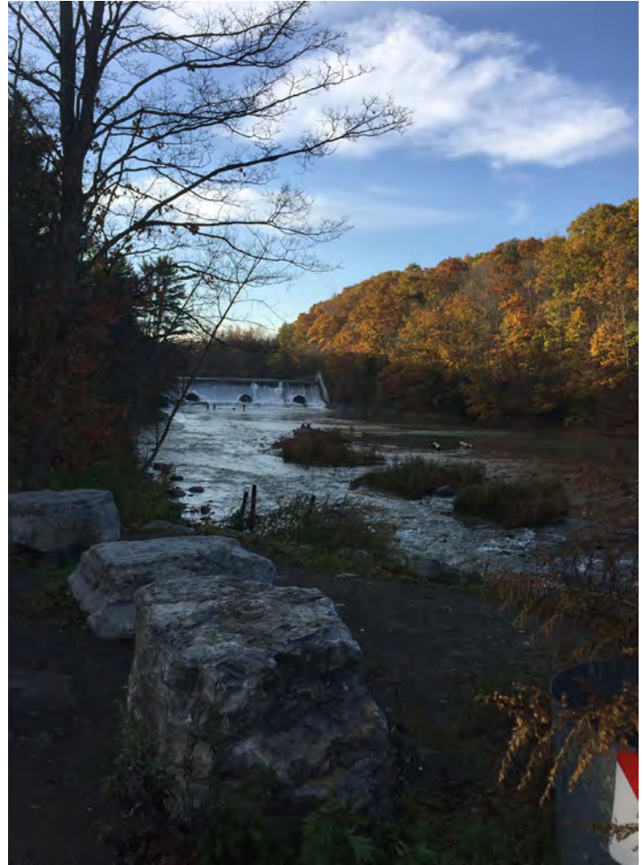
View of the dam from the parking area
