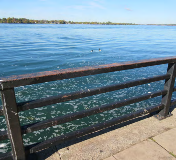
Railings need repairs and painting
