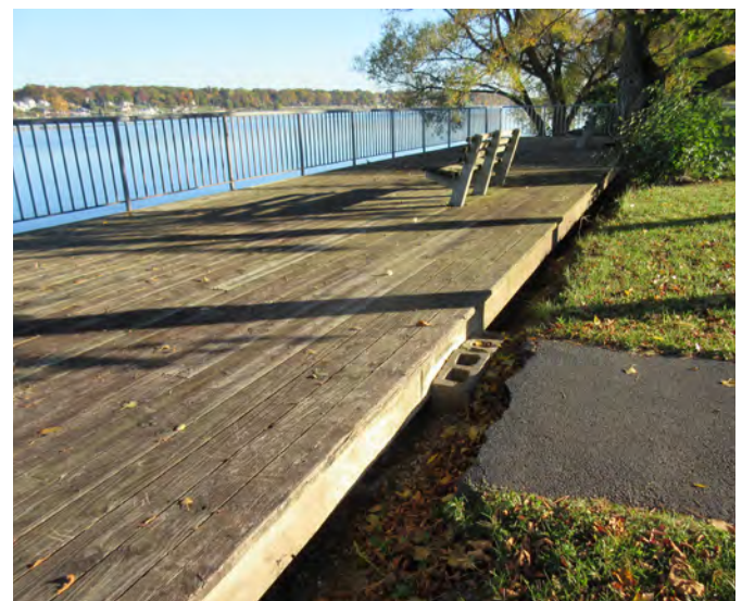
Section of asphalt path missing
