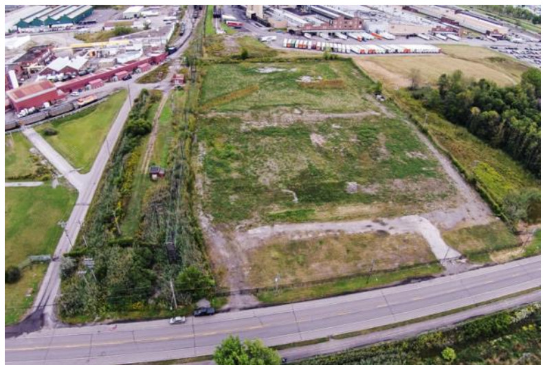
Polymer Applications Remediated Brownfield
