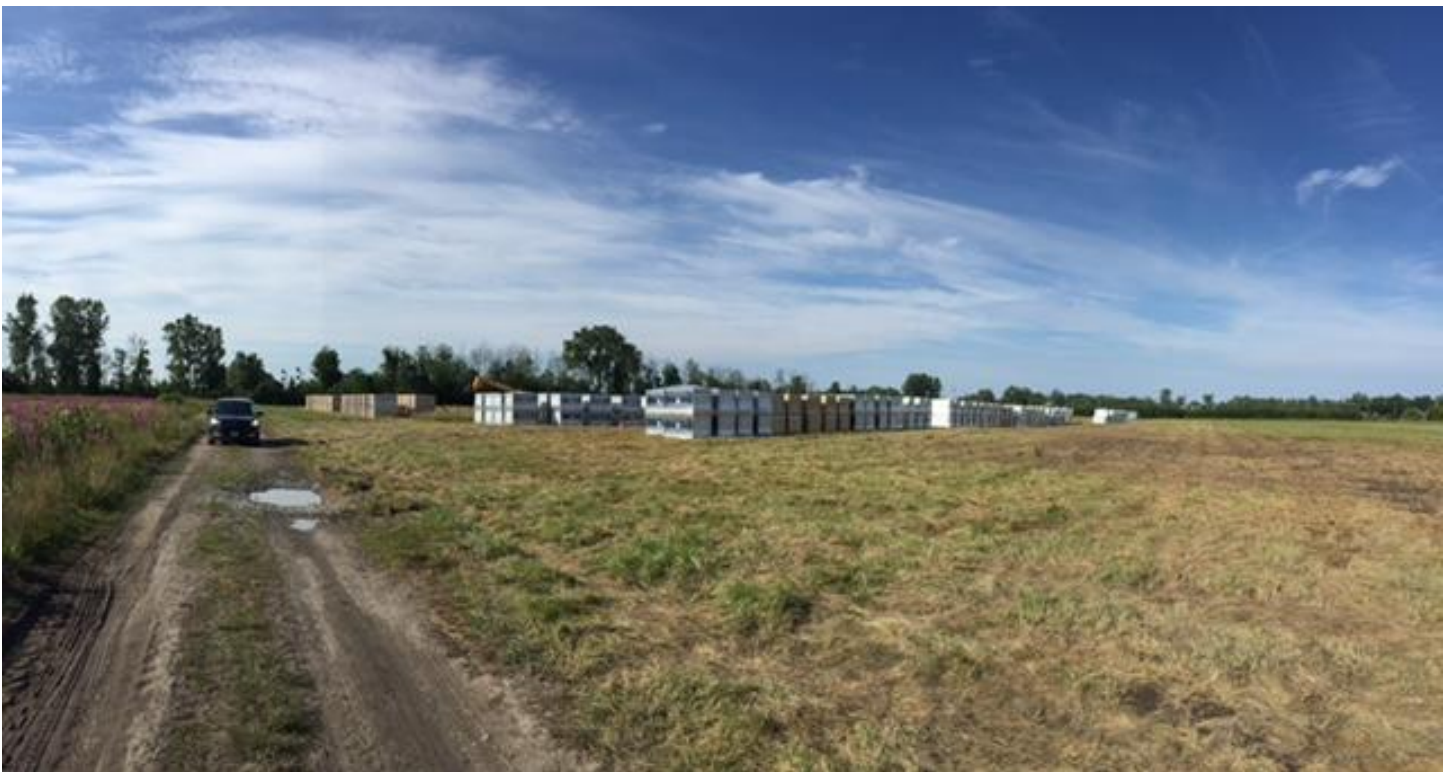
Site Preparation for Solar Panels at Erie County Correctional Facility
