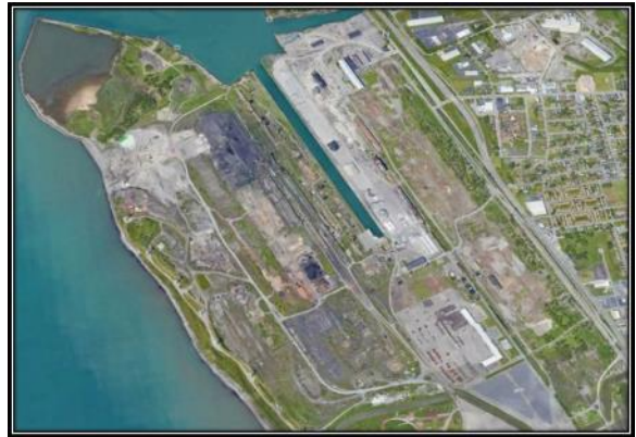
Aerial Photo of Bethlehem Steel
