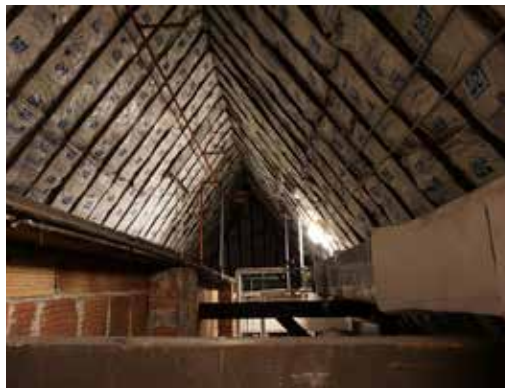
Insulation in Old County Hall
