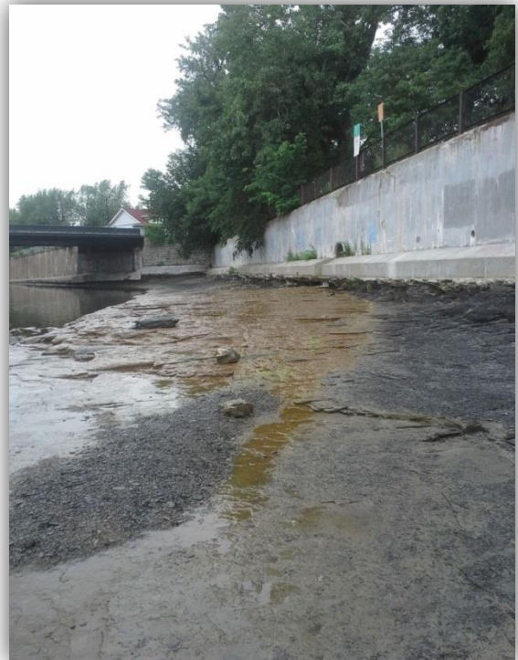
Figure 4.15: Combined Sewer Outfall, Cazenovia Creek
