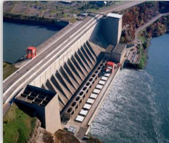
Figure 4.22: NYPA Hydroelectric Dam in Lewiston, NY
