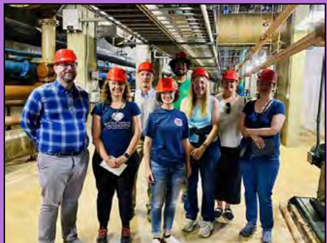
EMC Wastewater Treatment Facility Tour (From left to right: Jason Kulaszewski, Jeanne Beiter, Andrew Schrauth, Mayor Lynne Ruda, Marcus Rosten, Brenda Young, Bonnie Lawrence, Sharon Bachman)
