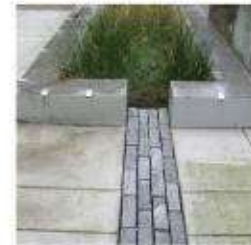
Open jointed paver water interception into a planted area
