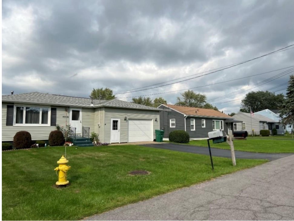
Photo 9: Residential structures on the north side of Roseview Avenue (4956 & 4962 Roseview Avenue), located north of the New Stadium.
