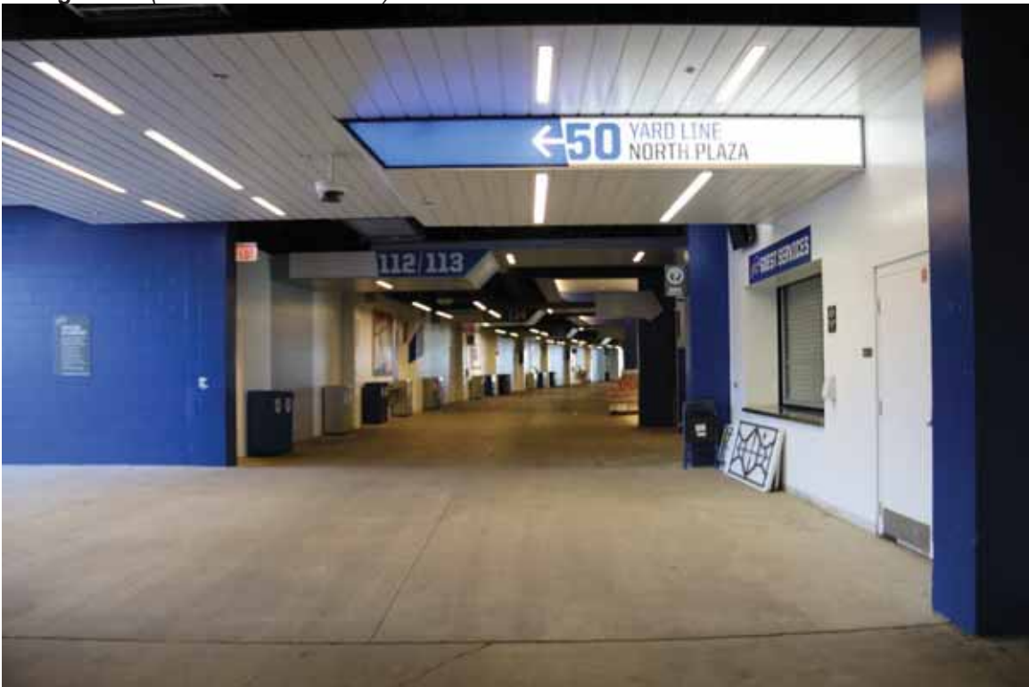
Photograph 56. 100 Level concourse at 50 Yard Line North South Plaza entrance (north sideline), facing east (Commonwealth 2022)
