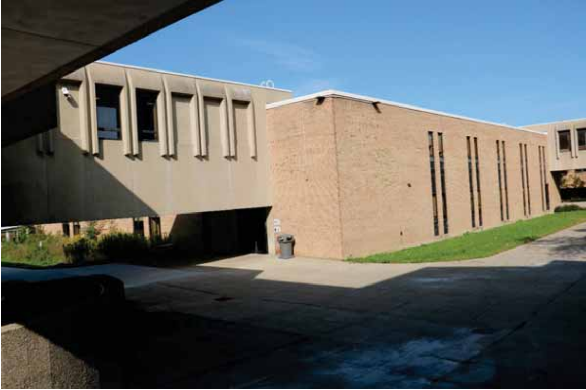
Photograph 23. Bridge 3-4 and Building 3, facing northwest ( Commonwealth 2022 ).
