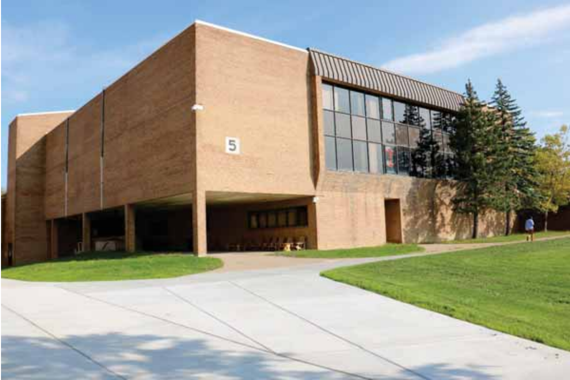
Photograph 29. Building 5, facing northeast ( Commonwealth 2022 ).
