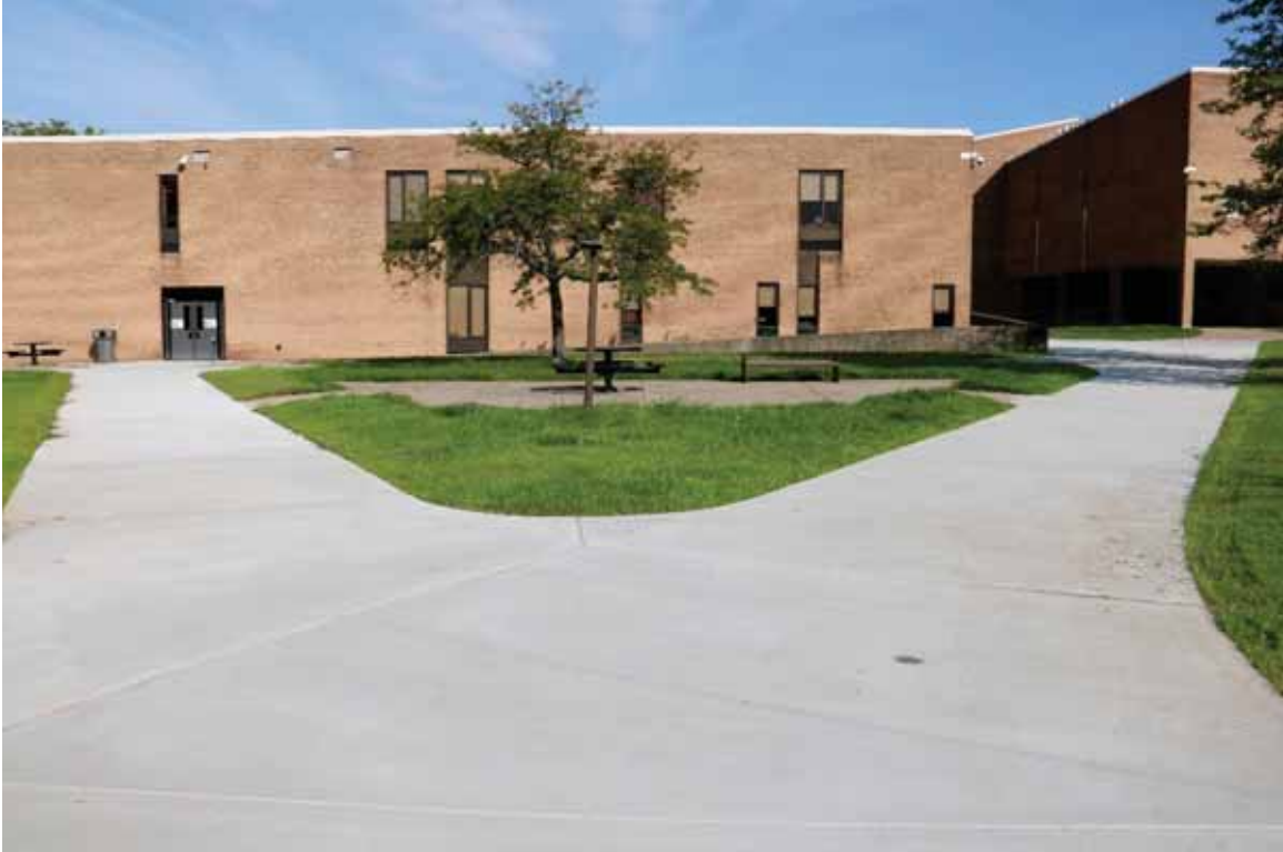
Photograph 27. Building 4 and southwest walkway to Main Court, facing north ( Commonwealth 2022 ).
