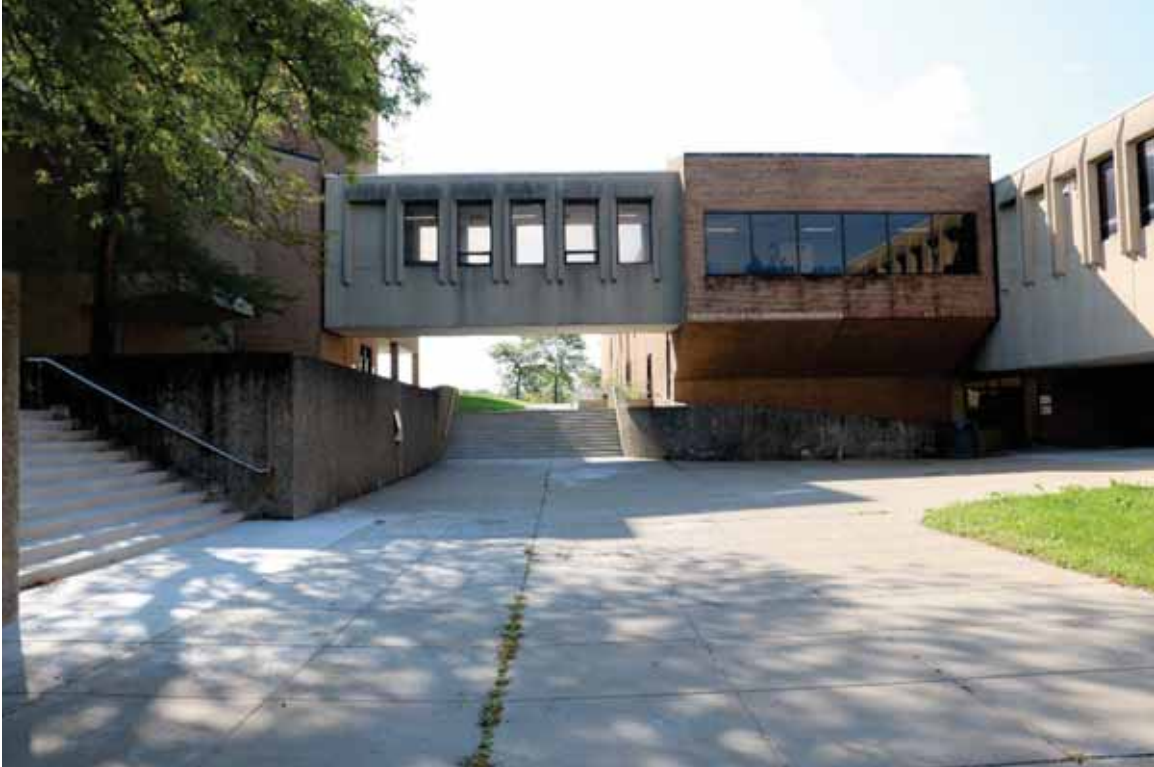
Photograph 31. Bridge 4-5 and north side of Building 4, facing south ( Commonwealth 2022 ).
