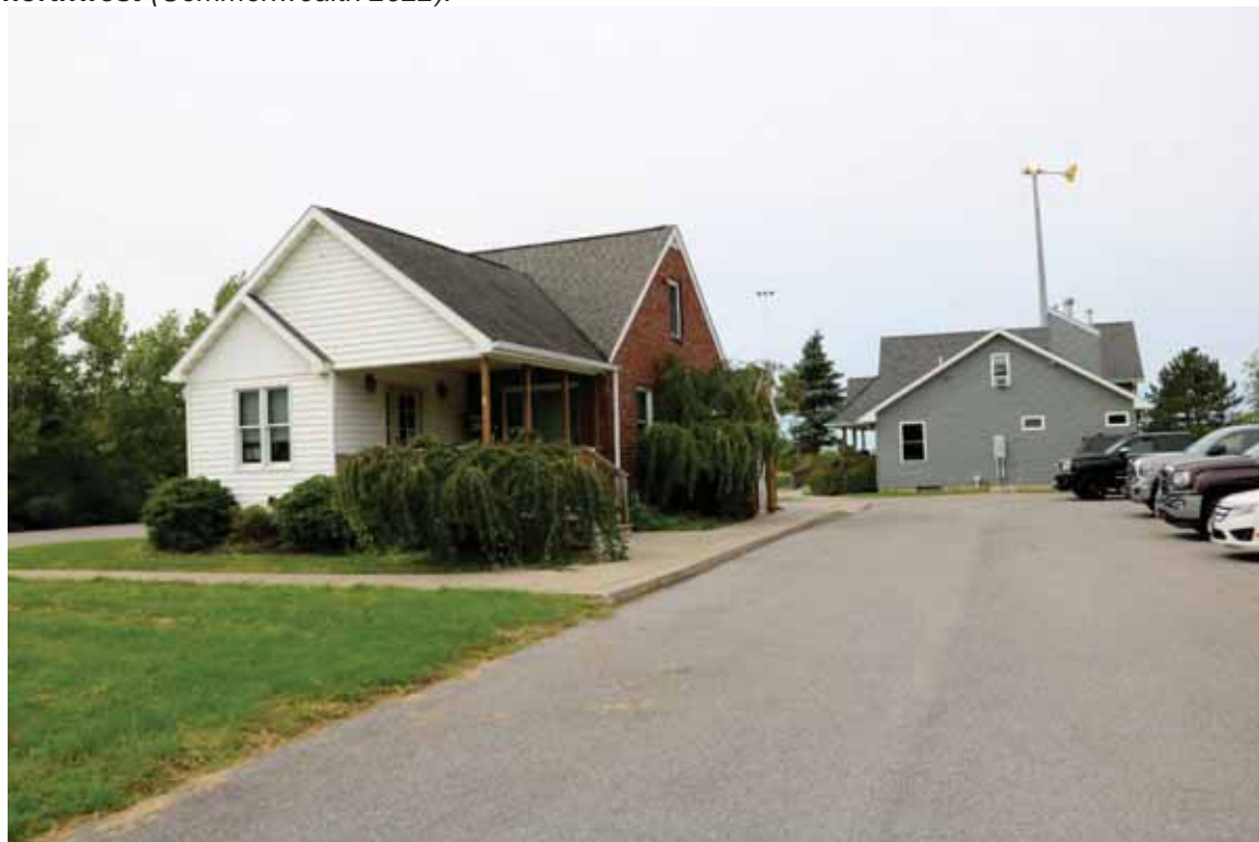
Photograph 48. SUNY Erie Green Building Technology Center (4196 Abbott Rd), facing northwest ( Commonwealth 2022 ).
