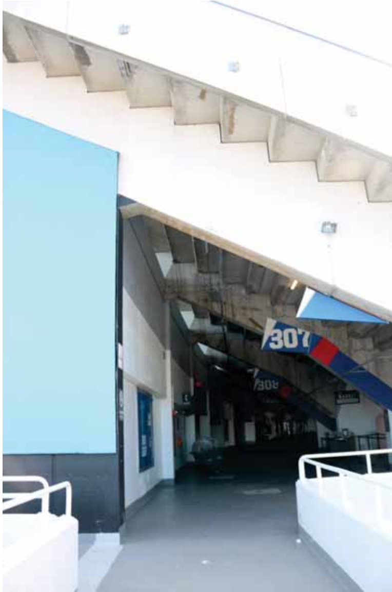
Photograph 73. 300 Level concourse entrance (north sideline), facing east (Commonwealth 2022).
