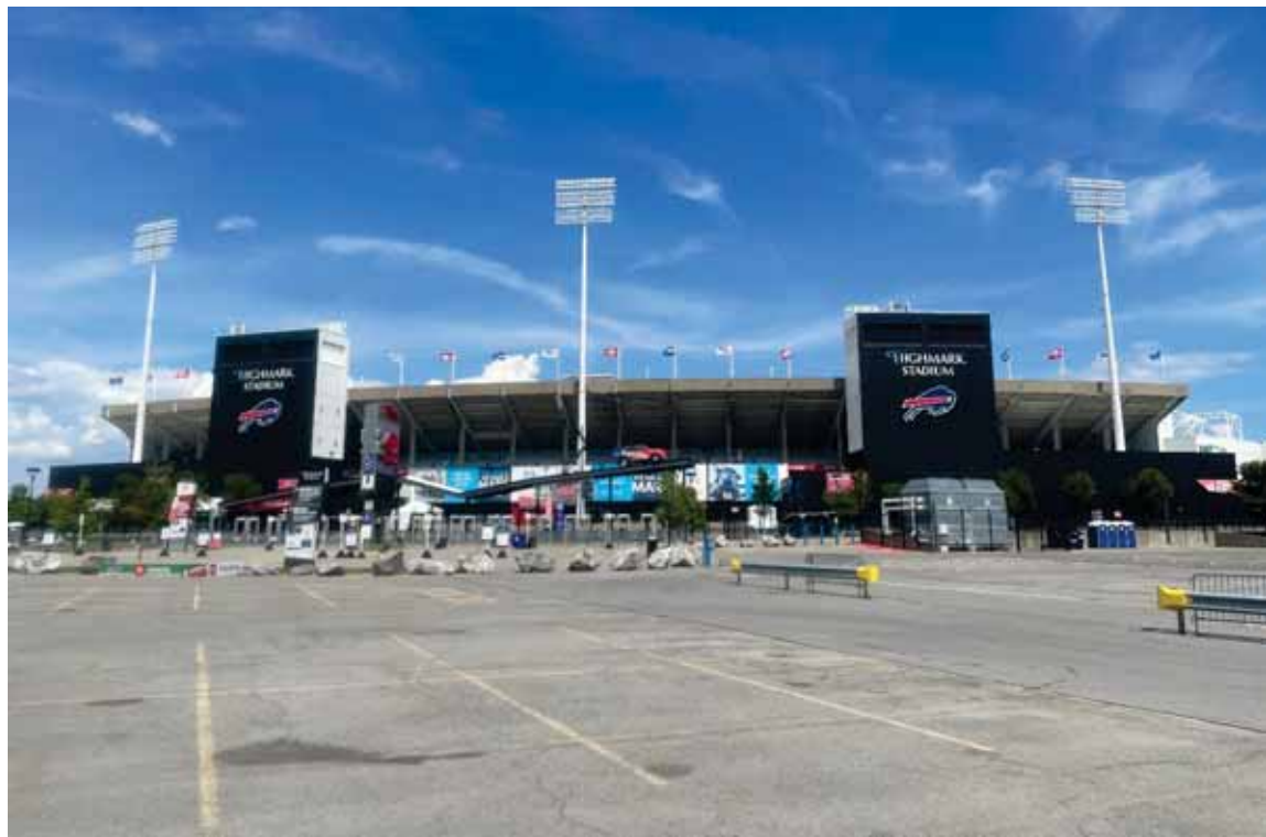
Photograph 2. South side of Highmark Stadium, facing north ( Commonwealth 2022 ).
