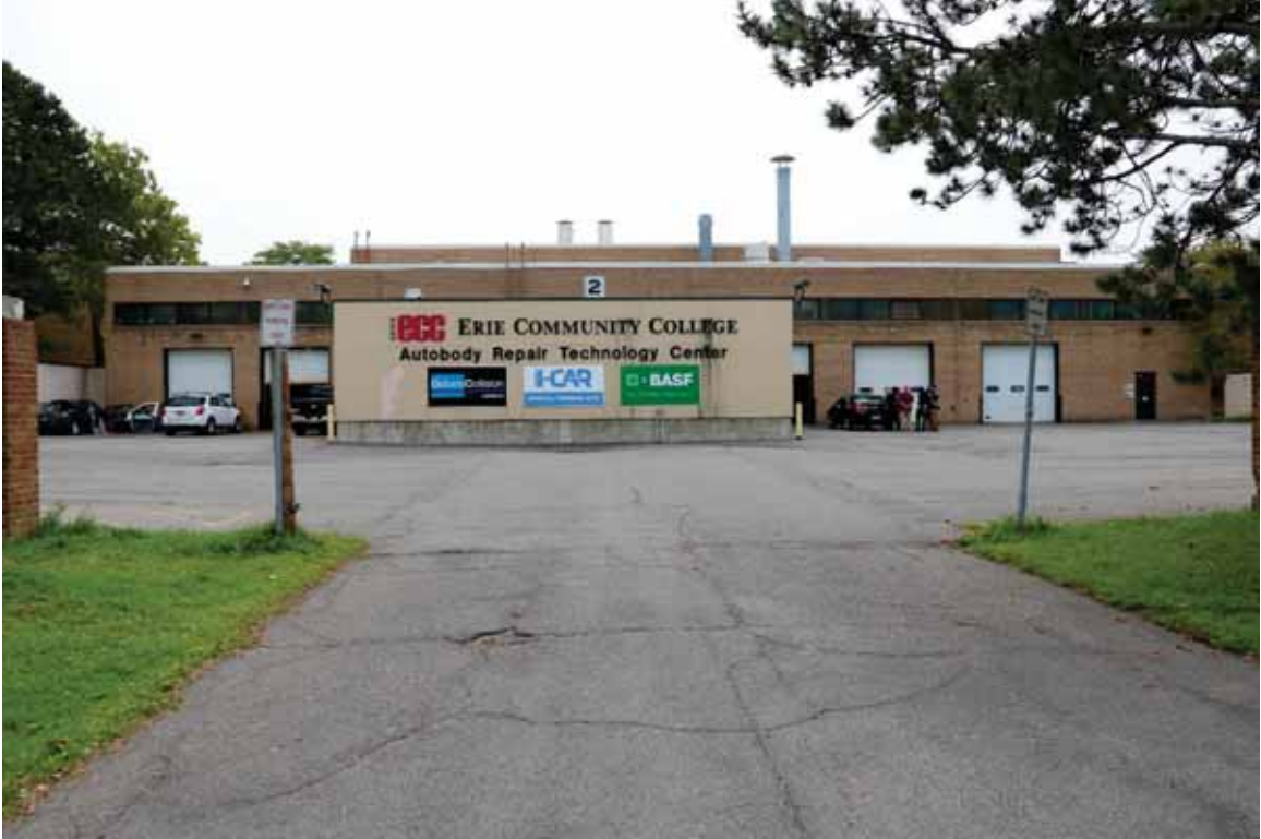
Photograph 17. North side of Building 2, facing south (Commonwealth 2022).
