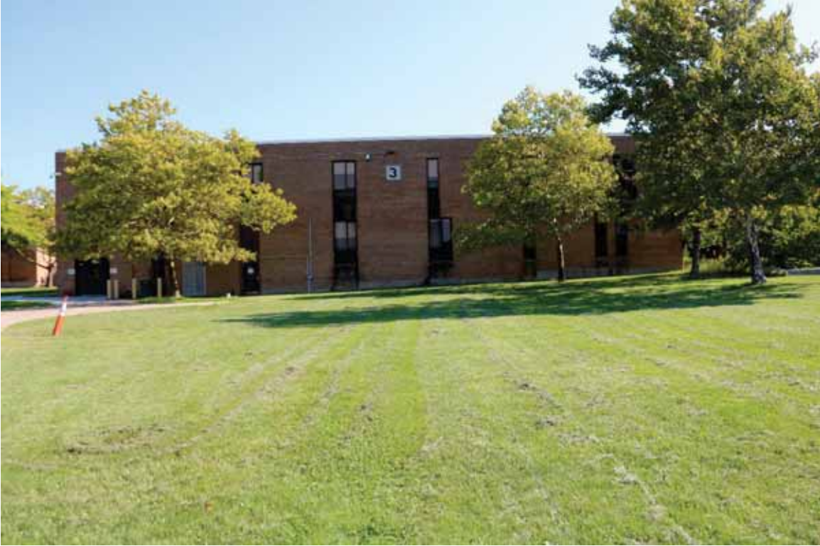
Photograph 25. Building 3, facing east ( Commonwealth 2022 ).
