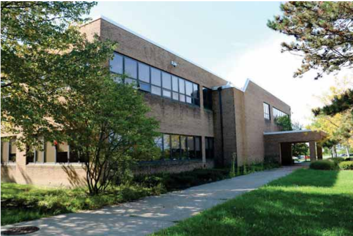
Photograph 12. North side of Building 1, facing southwest ( Commonwealth 2022 ).
