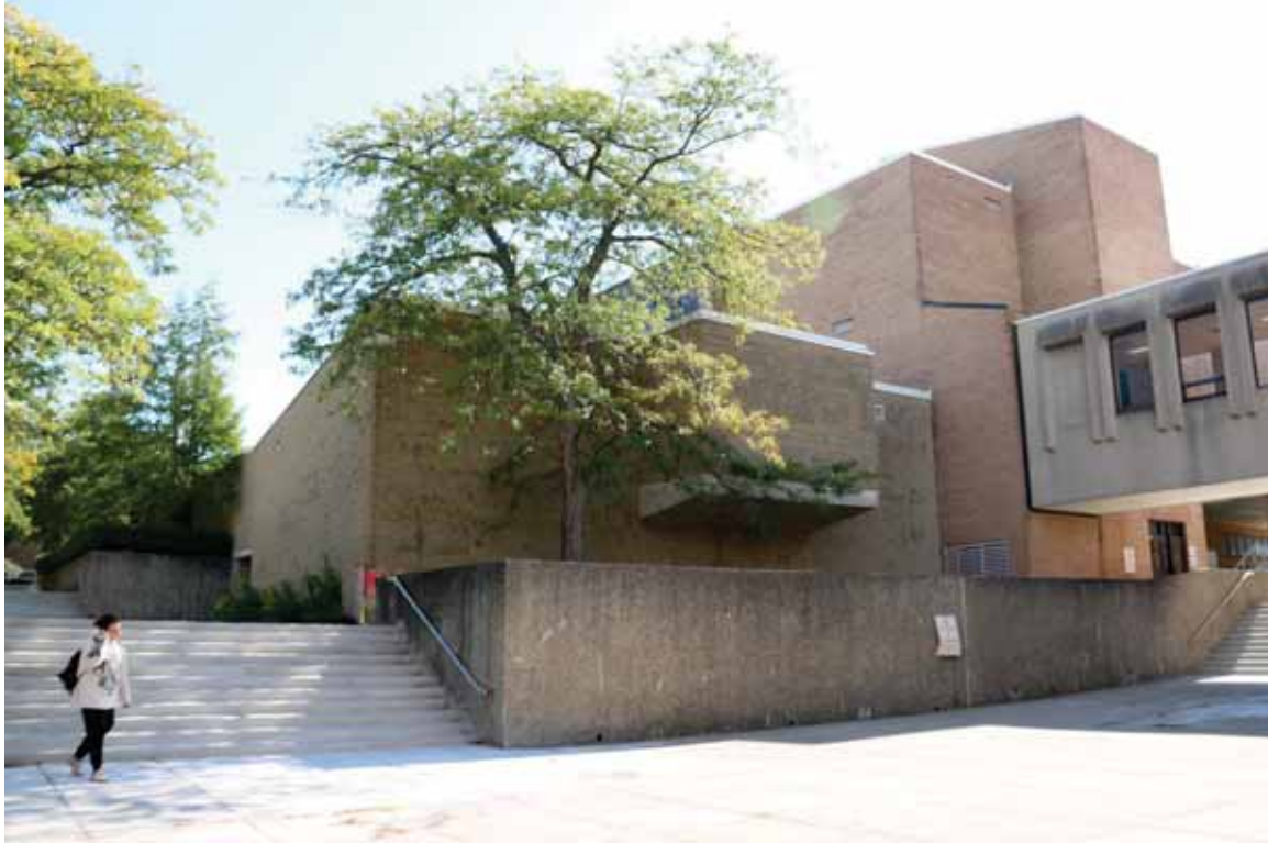
Photograph 33. Building 5, facing southeast ( Commonwealth 2022 ).
