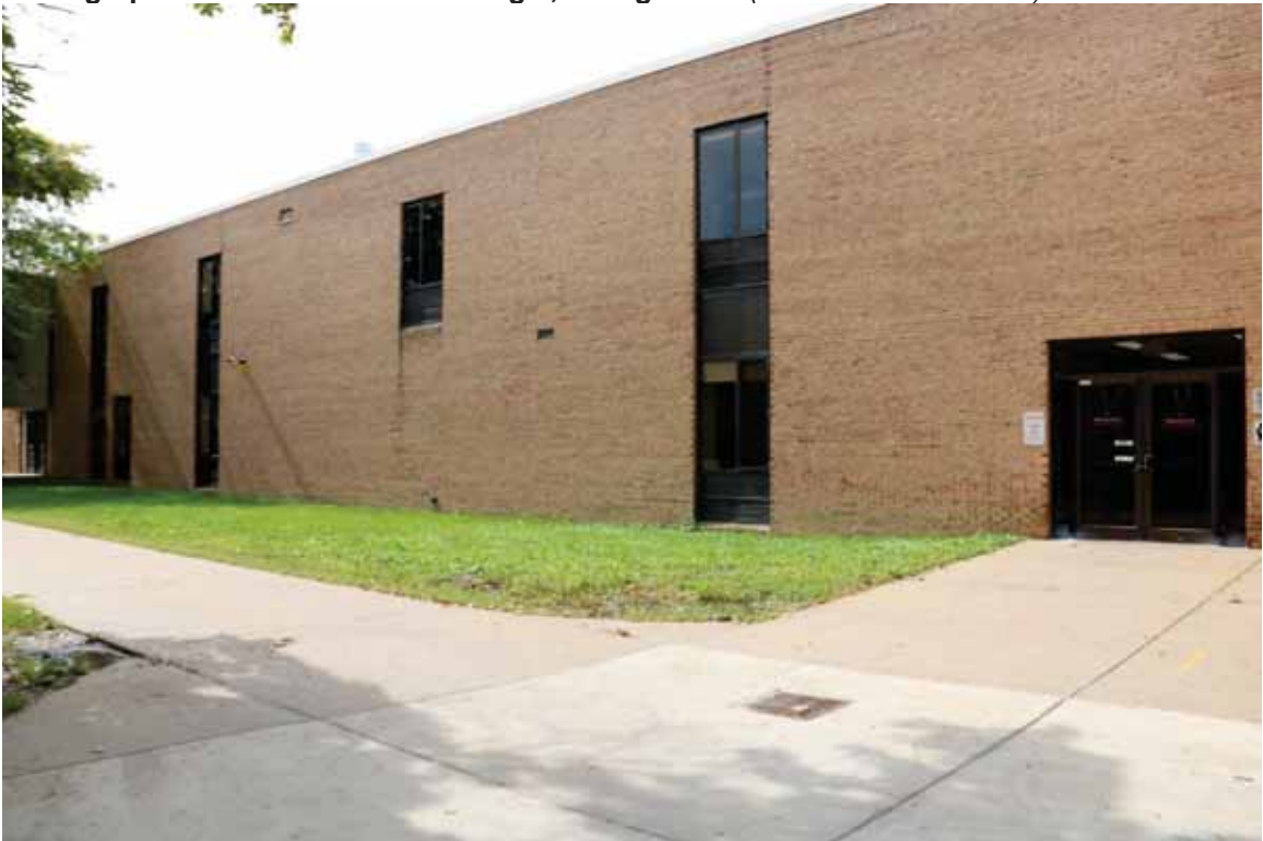
Photograph 18. East side of Building 2, facing southwest (Commonwealth 2022).
