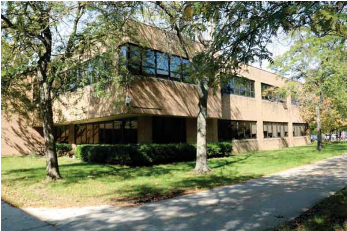
Photograph 14. South and east sides of Building 1, facing northwest ( Commonwealth 2022 ).
