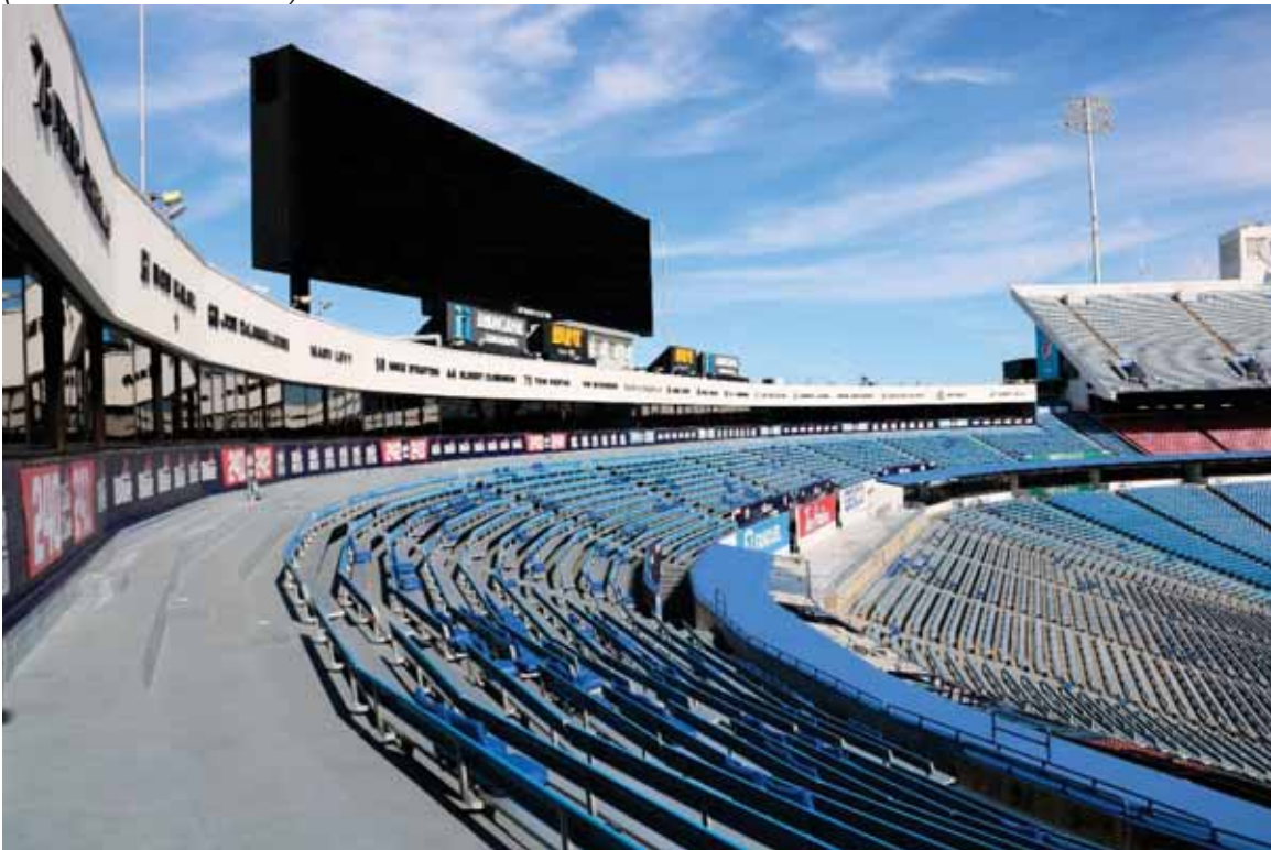
Photograph 41. 200 Level seating and main scoreboard in East End Zone, facing north (Commonwealth 2022).
