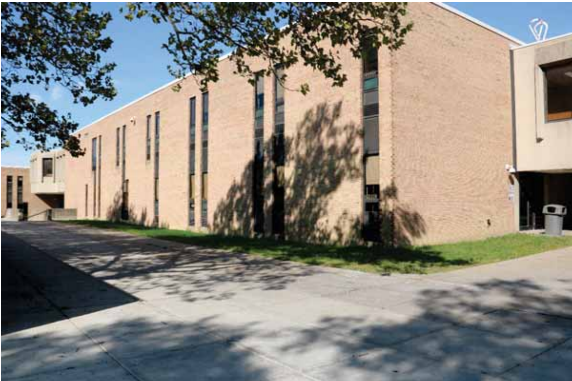
Photograph 20. Main Court side of Building 2, facing northwest ( Commonwealth 2022 ).
