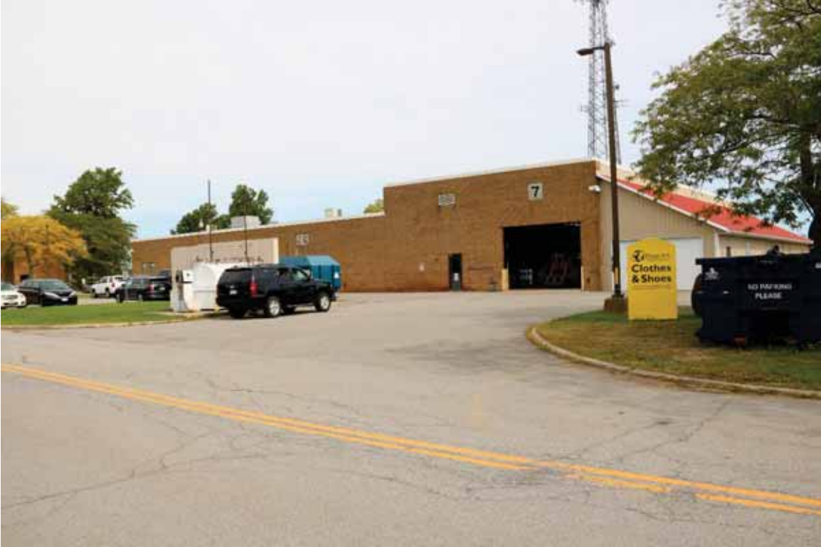
Photograph 45. Building 7, facing northeast (Commonwealth 2022).
