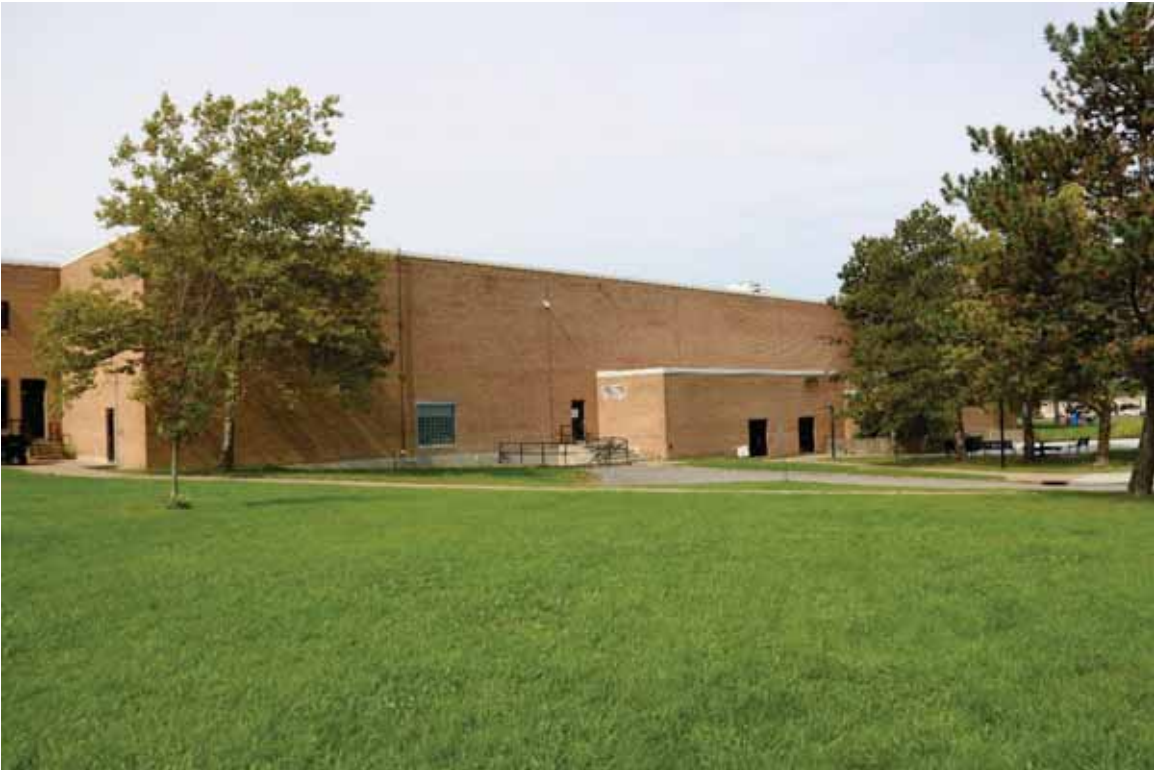
Photograph 42. Building 6, facing northwest ( Commonwealth 2022 ).
