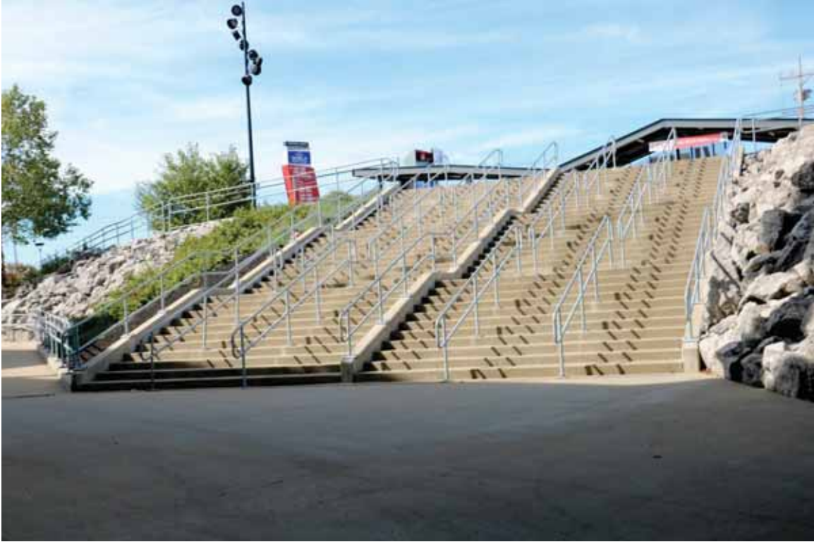
Photograph 5. West side of Highmark Stadium at Gate 4, facing west ( Commonwealth 2022 ).
