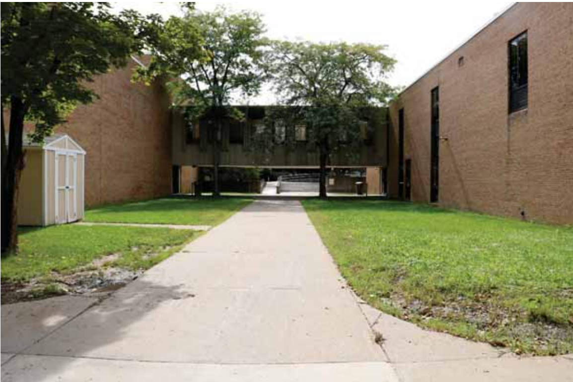
Photograph 44. Area between Buildings 2 and 6, facing south ( Commonwealth 2022 ).
