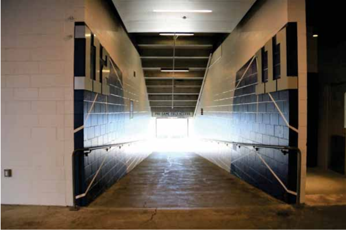
Photograph 59. 100 Level sideline (north) vomitory entrance from concourse (112/111), facing south (Commonwealth 2022).
