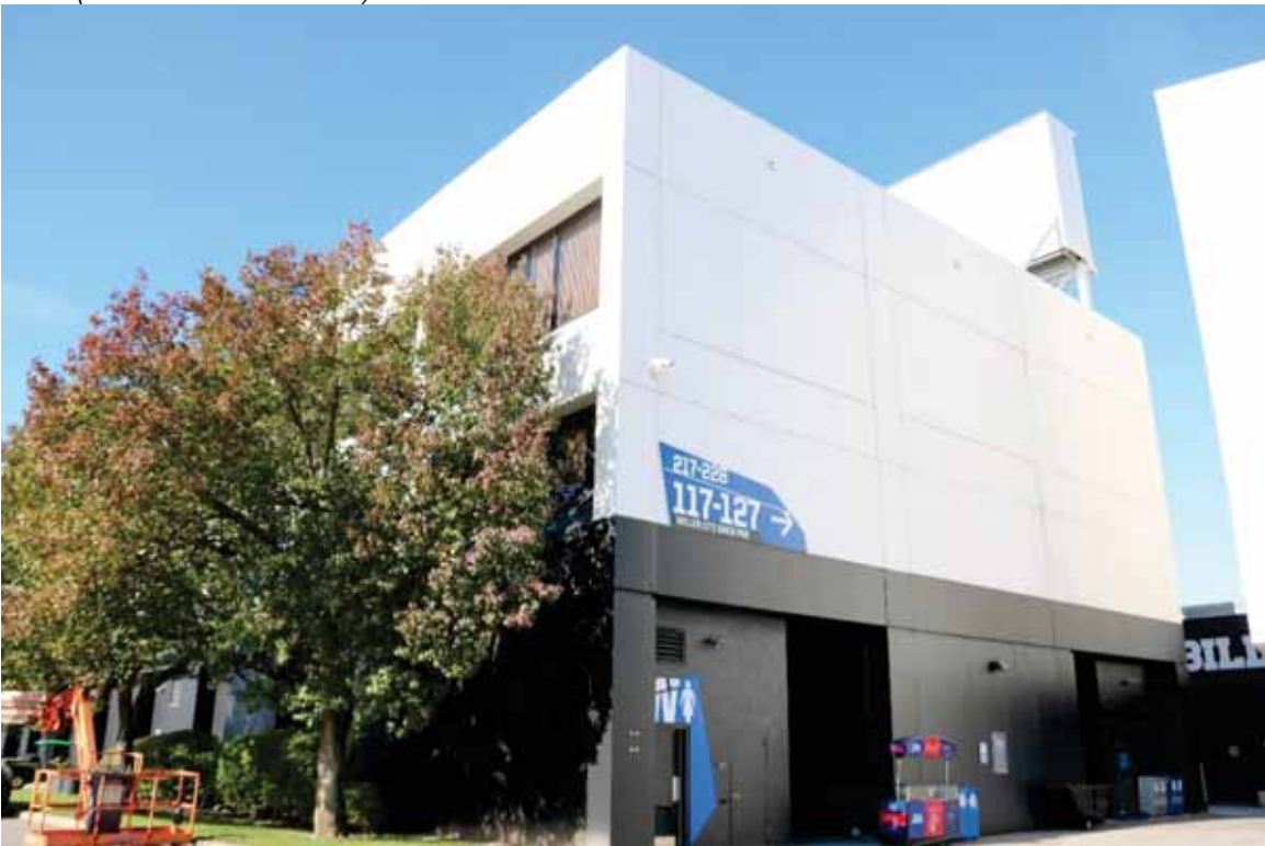
Photograph 14. East and north sides of Old Administration (Facilities) Building, facing southwest ( Commonwealth 2022 ).
