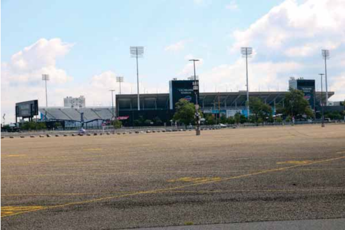
Photograph 1. Setting view of Highmark Stadium, facing northeast ( Commonwealth 2022 ).
