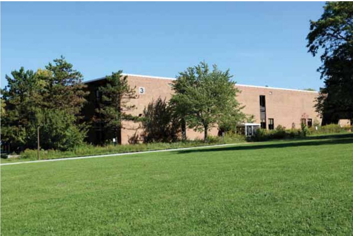
Photograph 24. Building 3, facing northeast ( Commonwealth 2022 ).
