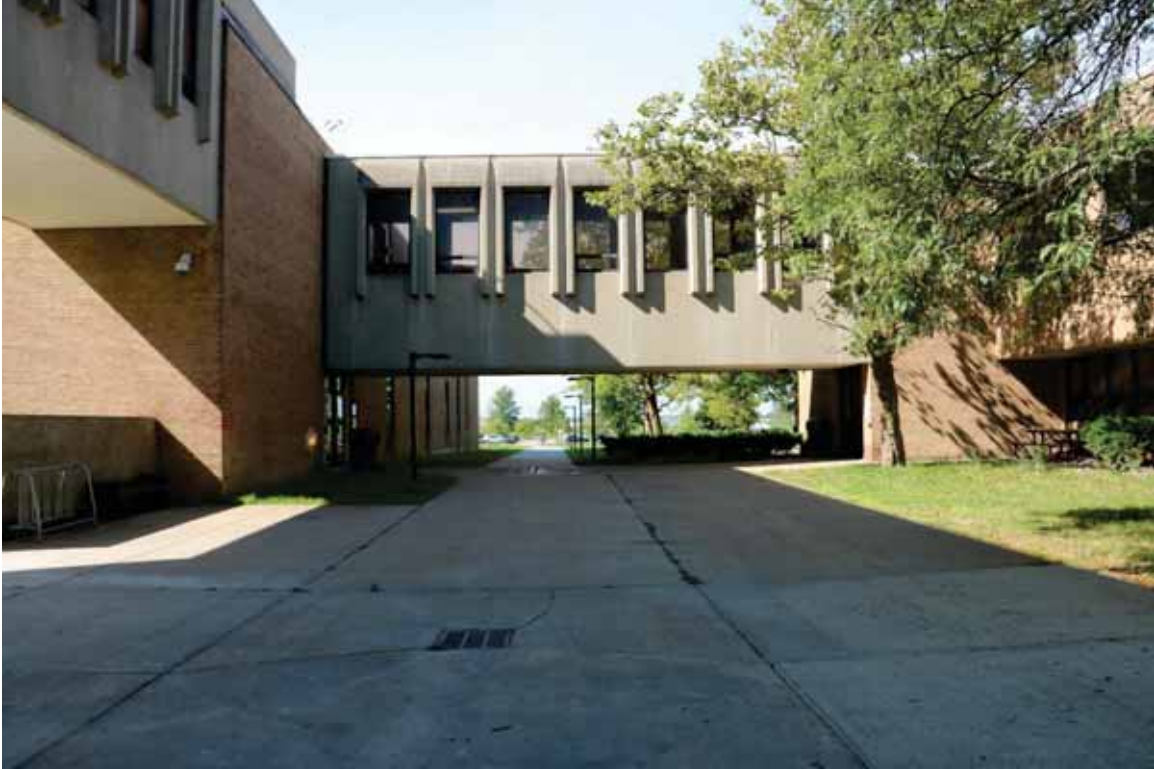
Photograph 15. Bridge 1-3 with Building 1 at right, facing west ( Commonwealth 2022 ).
