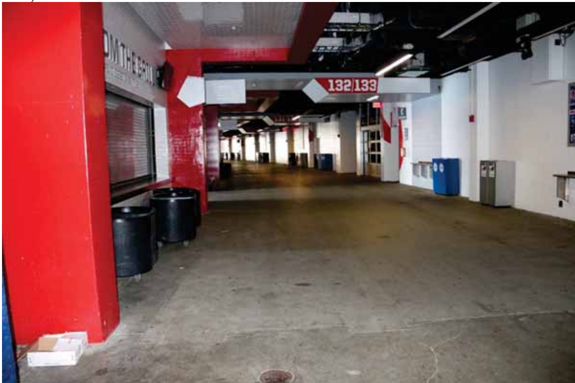
Photograph 54. 100 Level concourse example from 134/135 (south sideline), facing east ( Commonwealth 2022 ).
