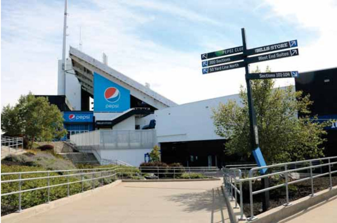
Photograph 7. Northwest entrance ramp, facing east (Commonwealth 2022).
