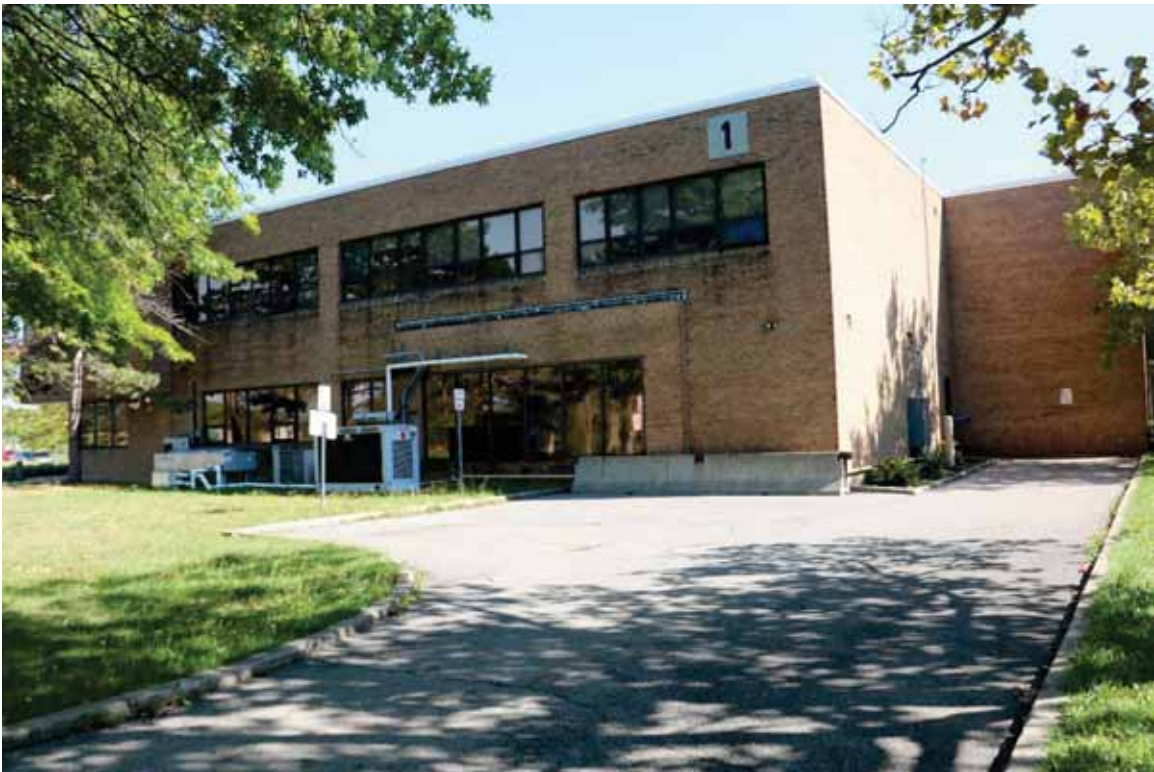
Photograph 16. West side of Building 1, facing northwest ( Commonwealth 2022 ).
