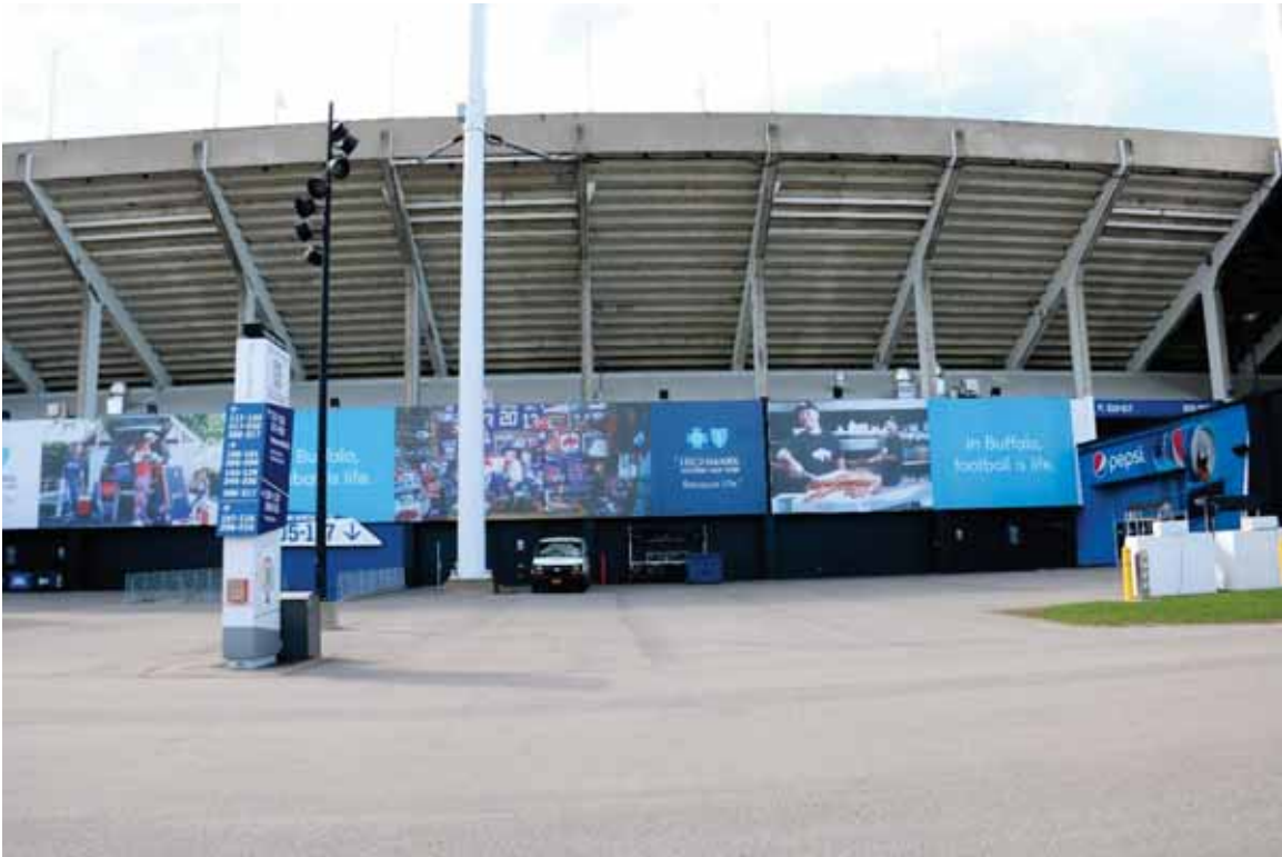
Photograph 11. 50 Yard Line North Plaza, facing south ( Commonwealth 2022 ).
