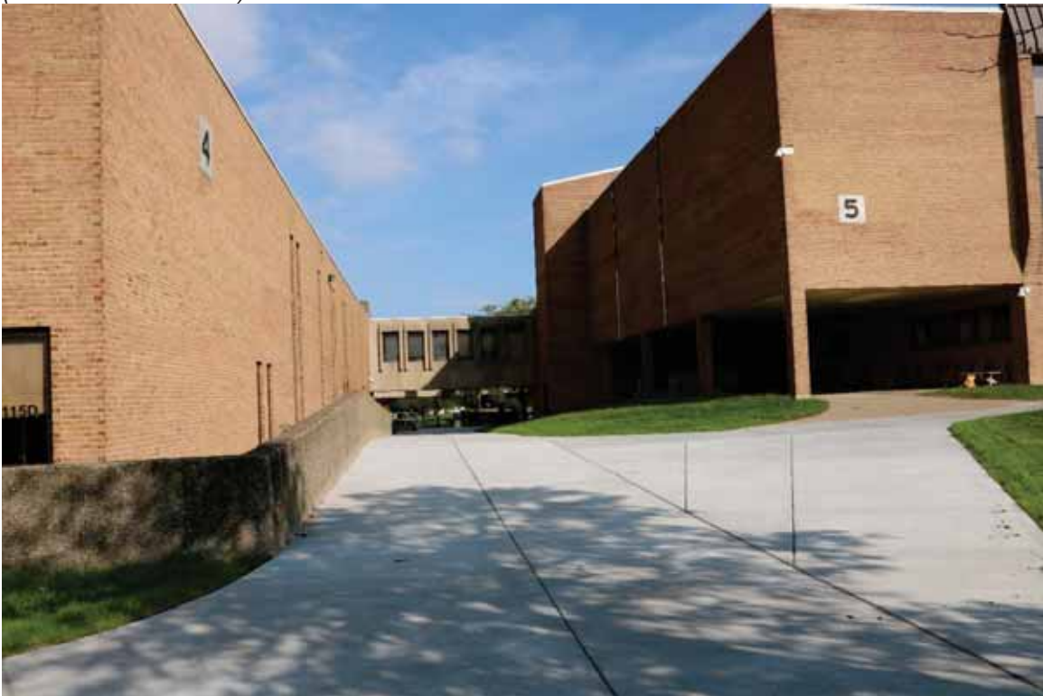
Photograph 28. Area between Buildings 4 and 5 with Bridge 4-5 and Main Court in distance, facing north ( Commonwealth 2022 ).
