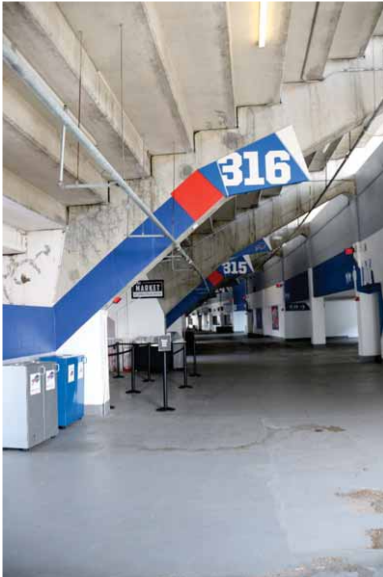
Photograph 74. 300 Level concourse (north sideline), facing west ( Commonwealth 2022 ).
