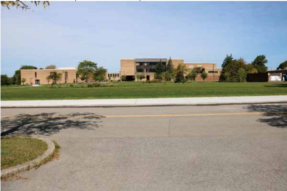
Photograph 6. Setting view of south side of SUNY Erie South Campus with Building 5 in center, facing north (Commonwealth 2022).
