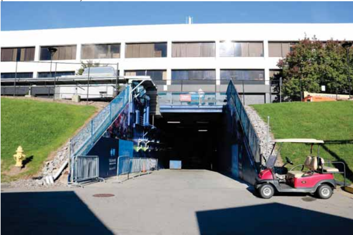
Photograph 16. East entrance to Tunnel at East End Zone, facing west (Commonwealth 2022).
