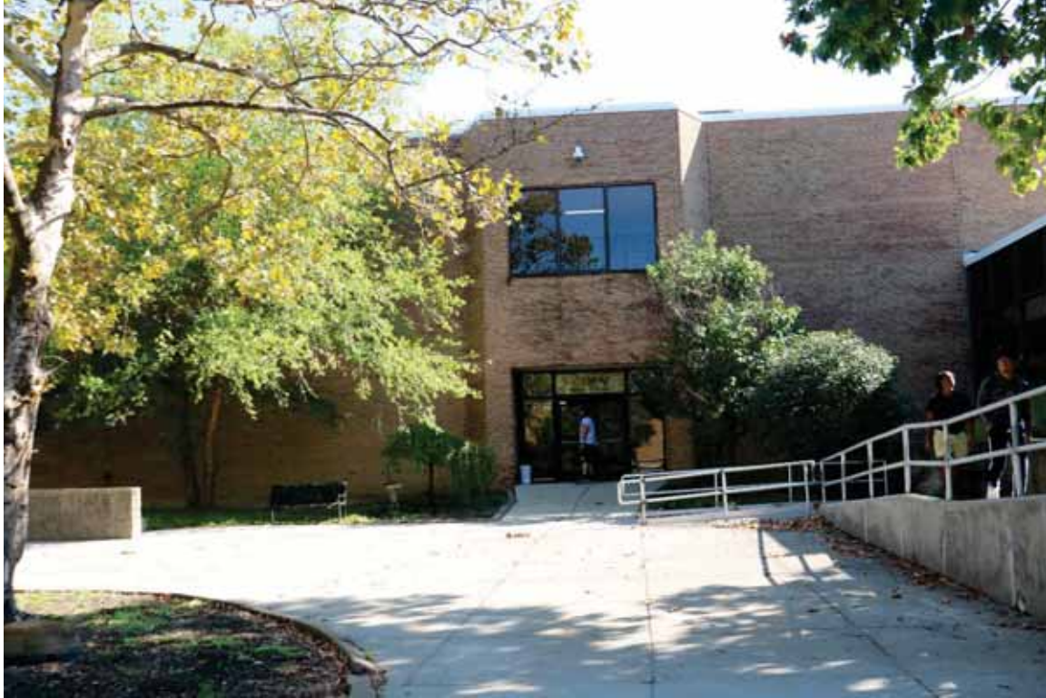
Photograph 39. Building 6, facing east ( Commonwealth 2022 ).
