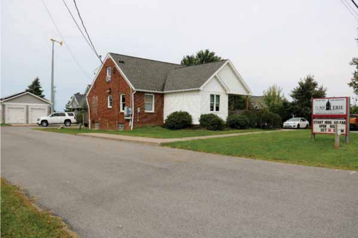
Photograph 47. SUNY Erie Green Building Technology Center (4196 Abbott Rd), facing northwest ( Commonwealth 2022 ).
