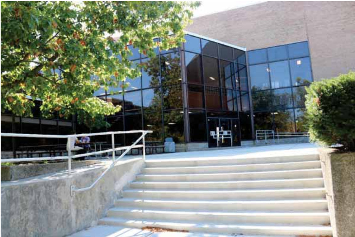
Photograph 38. Building 5, facing southeast ( Commonwealth 2022 ).
