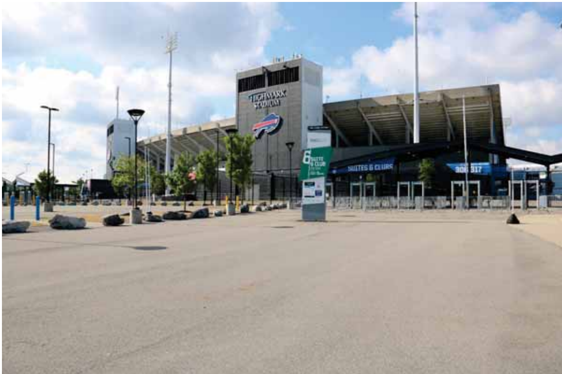
Photograph 8. North side of Highmark Stadium, facing southeast (Commonwealth 2022).
