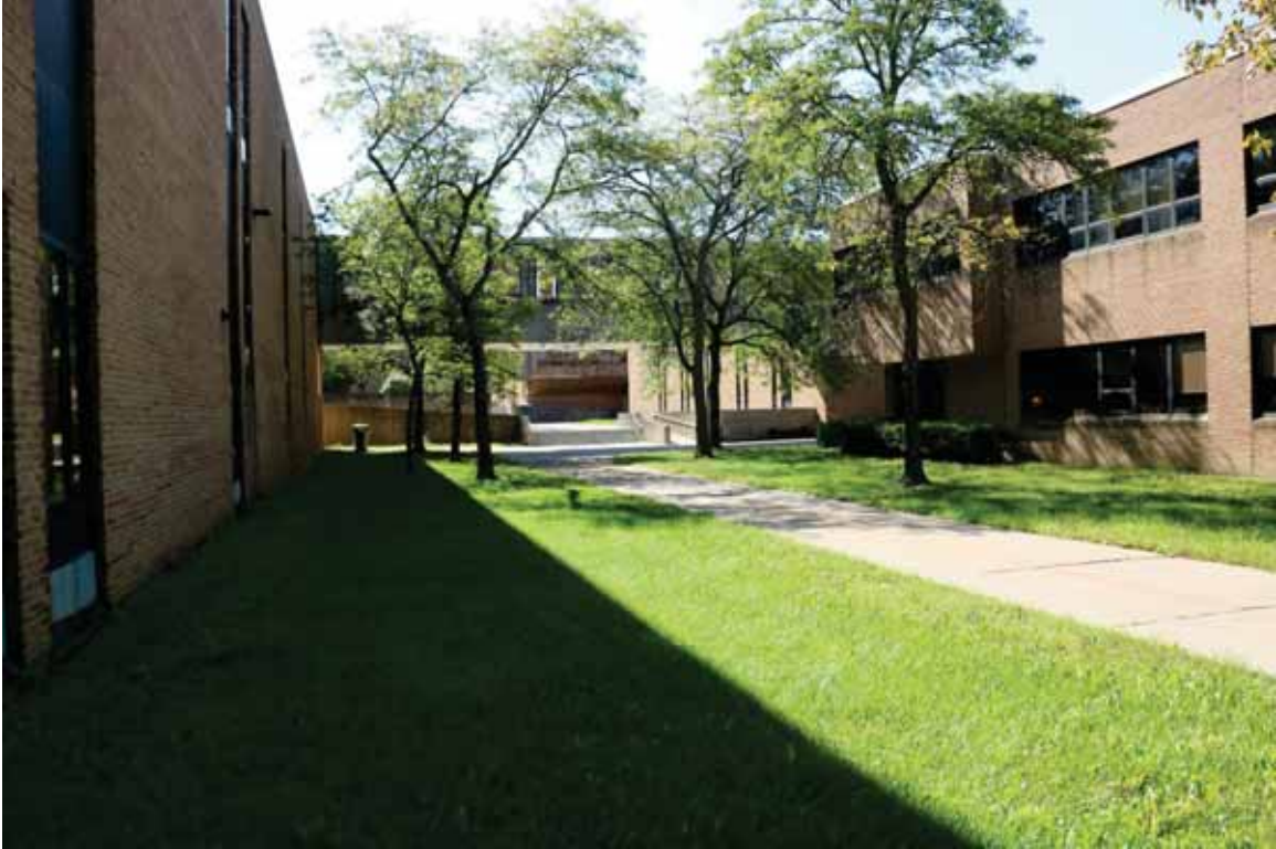
Photograph 13. Area between Buildings 1 (at right) and 2 with Bridge 2-3 and Main Court in background, facing south ( Commonwealth 2022 ).
