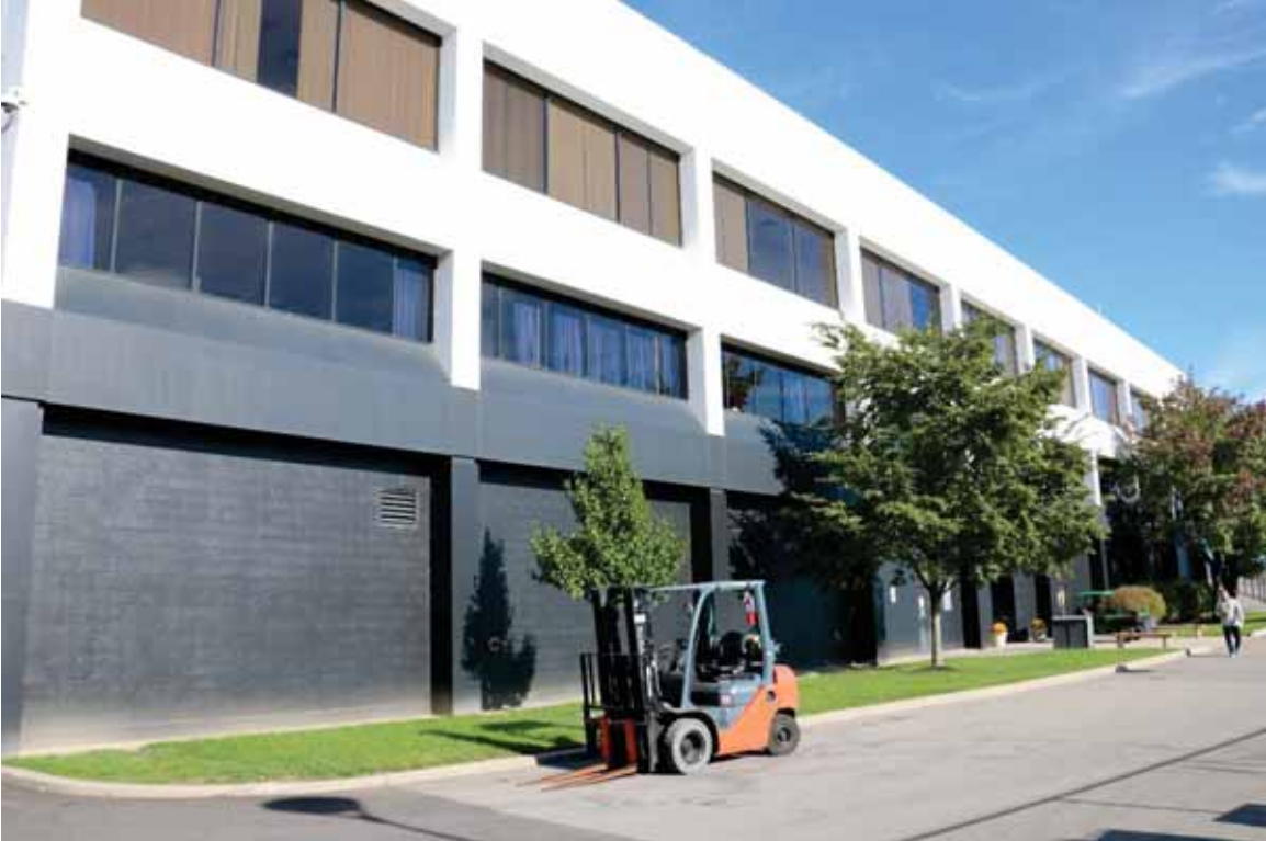
Photograph 15. East side of Old Administration (Facilities) Building, facing northwest (Commonwealth 2022).
