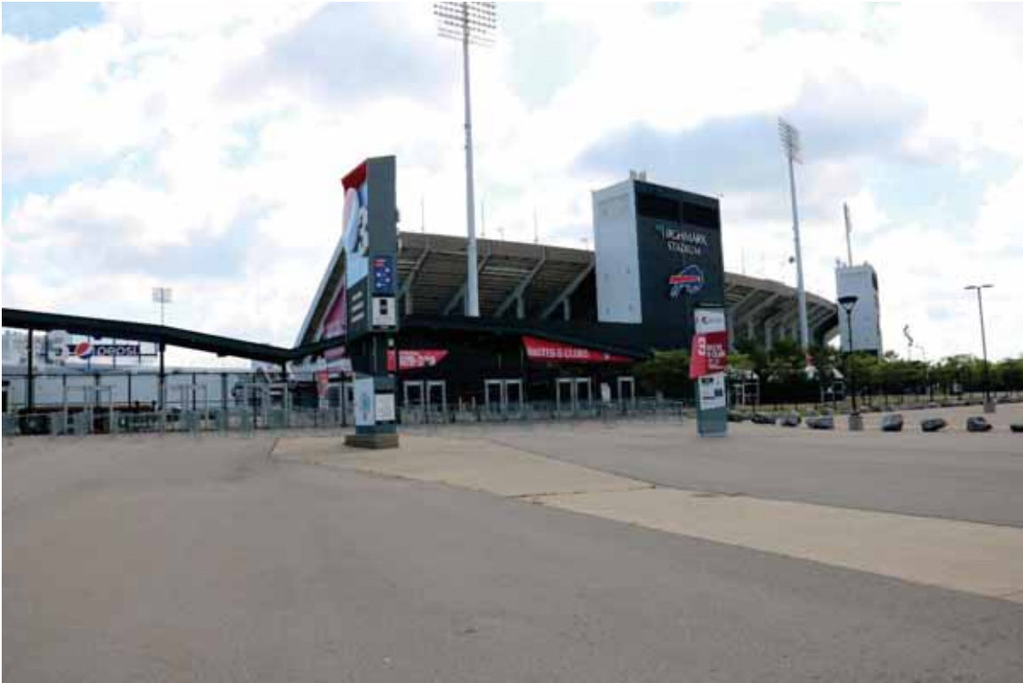
Photograph 3. South side of Highmark Stadium, facing northeast ( Commonwealth 2022 ).
