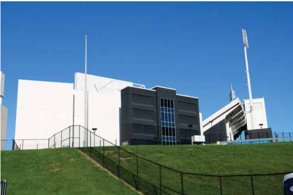
Photograph 12. Northeast section of Highmark Stadium, facing west ( Commonwealth 2022 ).
