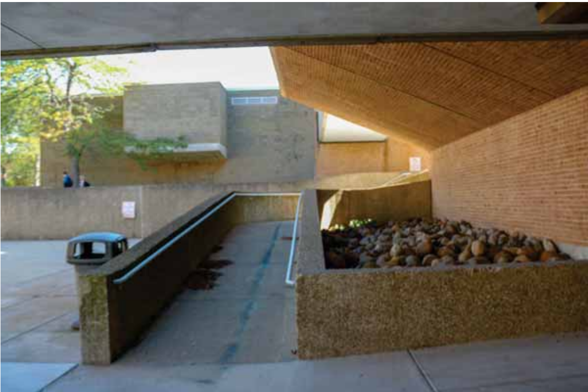
Photograph 32. Building 4 ramp, facing east ( Commonwealth 2022 ).
