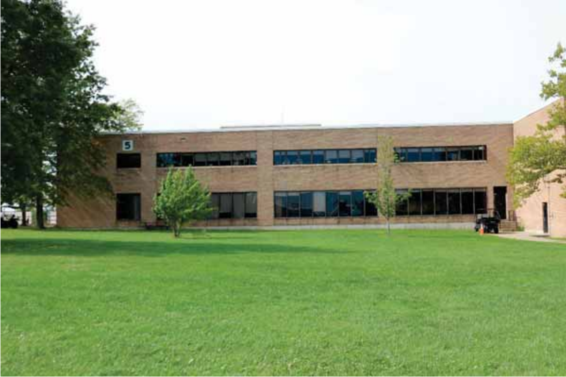
Photograph 41. Building 5, facing west ( Commonwealth 2022 ).
