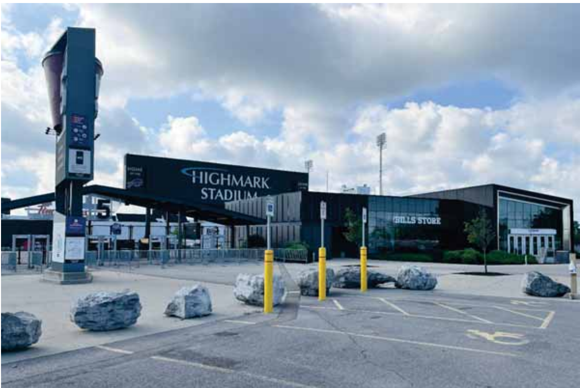
Photograph 4. West side of Highmark Stadium at Gate 5 with Bills Store at right, facing southeast ( Commonwealth 2022 ).
