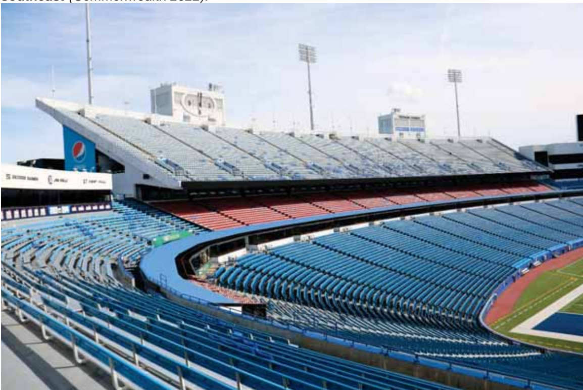
Photograph 45. View of south sideline seating from 200 Level of East End Zone, facing southeast (Commonwealth 2022).
