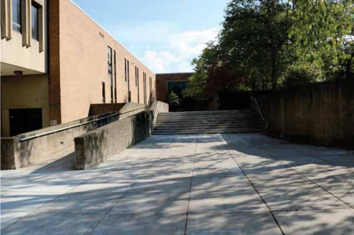
Photograph 21. Main Court side of Building 2, facing west ( Commonwealth 2022 ).
