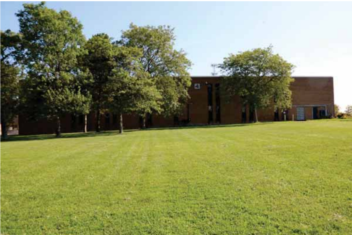
Photograph 26. Building 4, facing east ( Commonwealth 2022 ).
