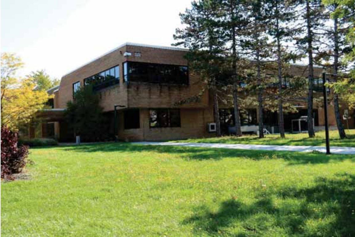
Photograph 9. Building 1, facing southeast ( Commonwealth 2022 ).
