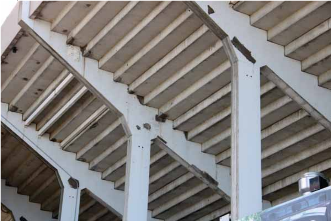
Photograph 10. Construction detail of 300 Level north, facing southeast ( Commonwealth 2022 ).
