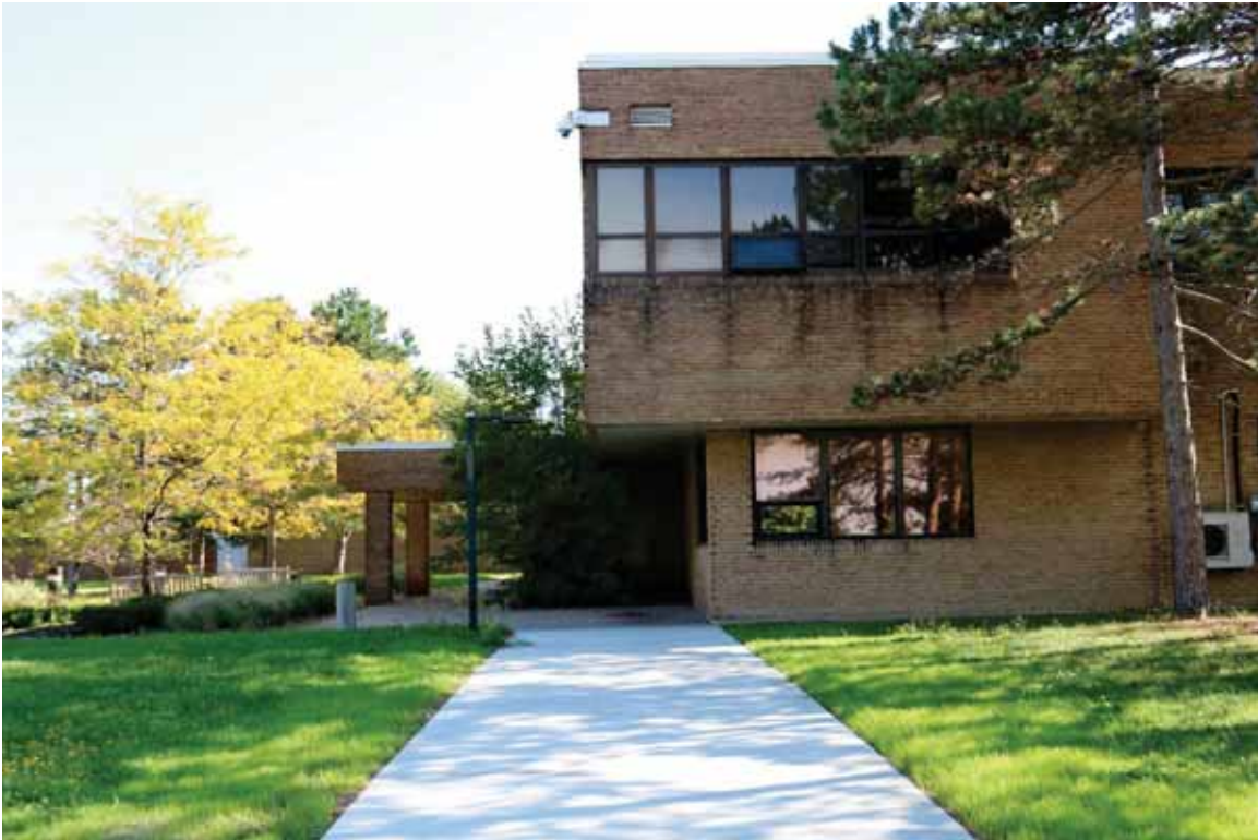
Photograph 10. Building 1 with north entrance in center, facing east ( Commonwealth 2022 ).
