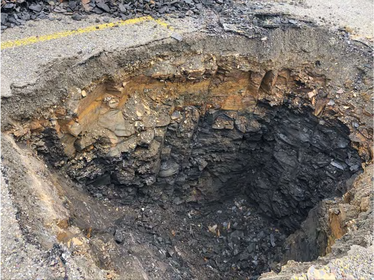
TEST PIT TP-2-22. Test pit excavated to a depth of approximately 10.0 feet. Weathered rock transitions to competent rock at approximately 9.2 feet.
