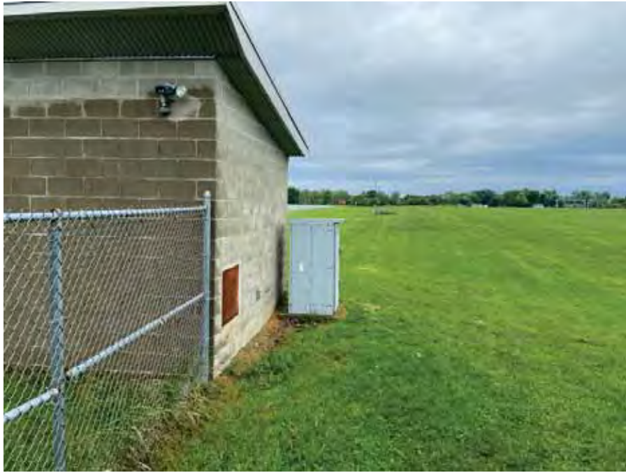
Photo 125 : Typical exterior of Building Nine
