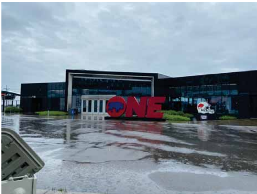
Photo 70 : Eastern exterior of Building Three
