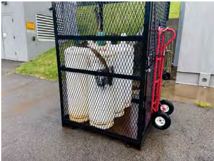
Photo 58 : Argon and Nitrogen containers located east of Building One
