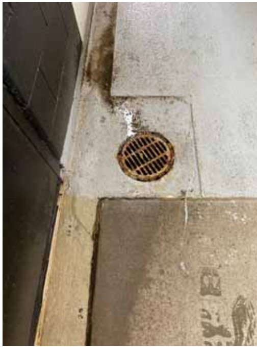
Photo 37 : Typical floor drain within Building One
