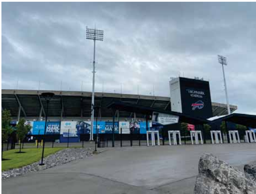
Photo 6 : Northern exterior of Building One
