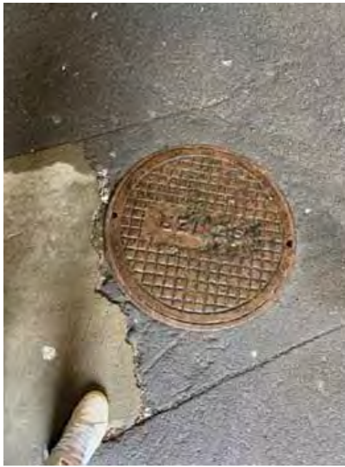
Photo 33 : Sewer outlet within Building One
