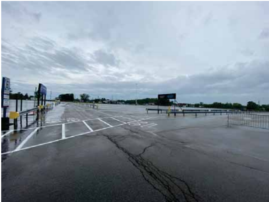
Photo 102 : Typical parking lot area
