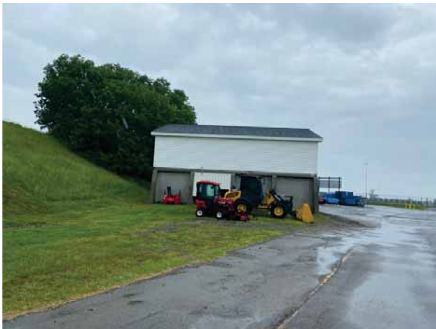
Photo 88 : Southern exterior of Building Five
