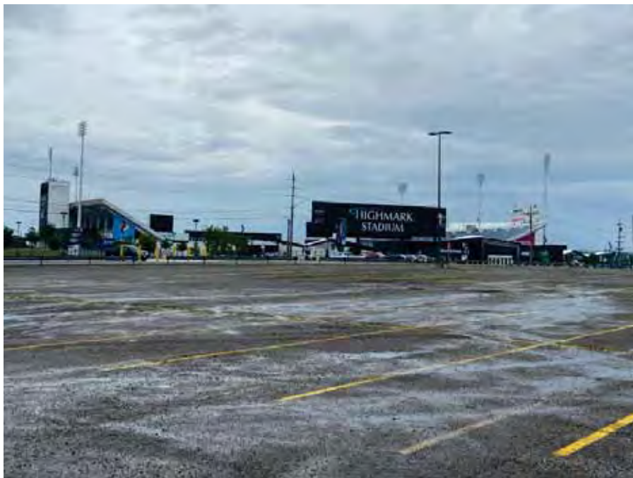
Photo 4 : Northern exterior of Building One
