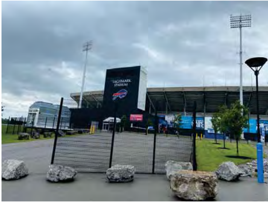
Photo 5 : Northern exterior of Building One
