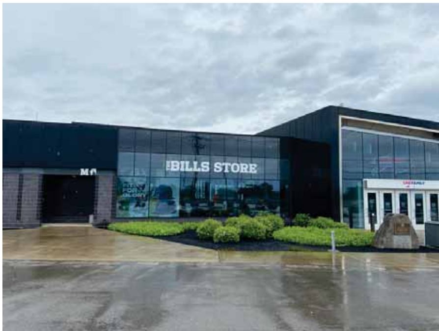
Photo 72 : Eastern exterior of Building Three
