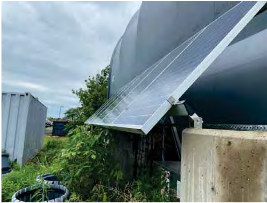
Photo 113 : Southern exterior of Building Eight
