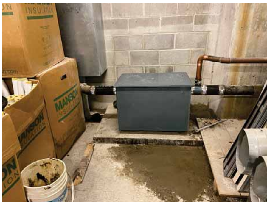
Photo 30 : Typical grease trap in Building One in Concession Area
