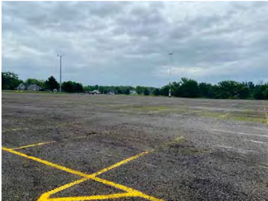
Photo 98 : Typical parking lot area across from Abbott Road
