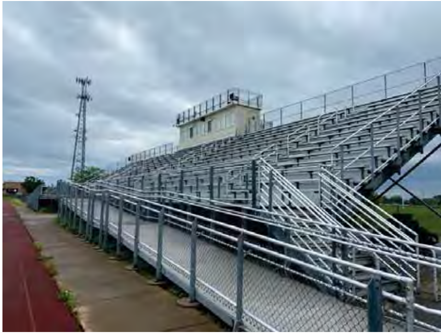
Photo 131 : Bleachers on ECC campus in Area Two
