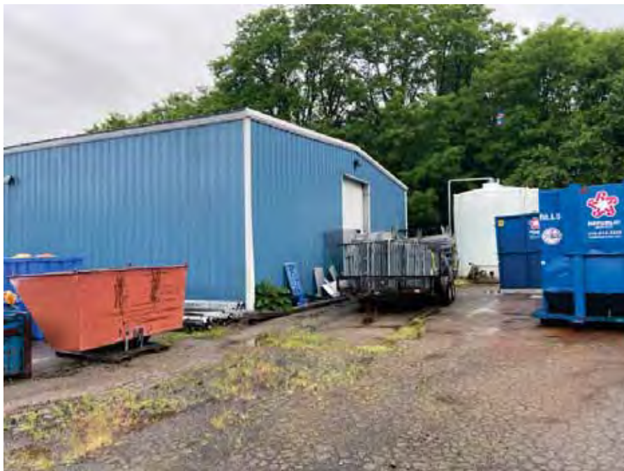
Photo 78 : Northern exterior of Building Four
