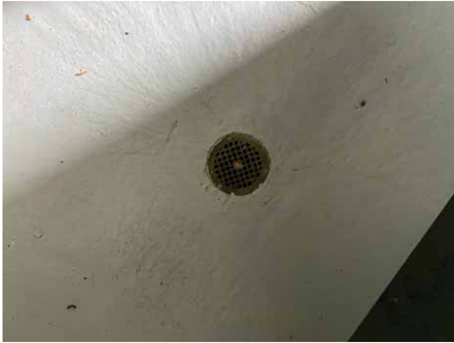
Photo 127 : Floor drain in Building Nine
