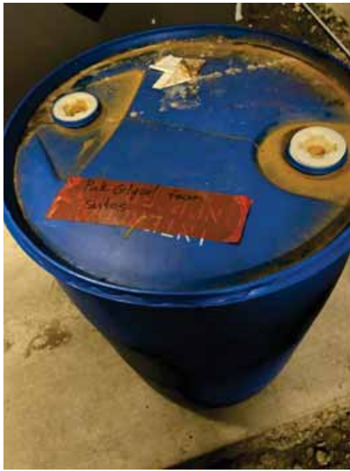
Photo 45 : 55-gallon drum of Pink Glycol in Building One
