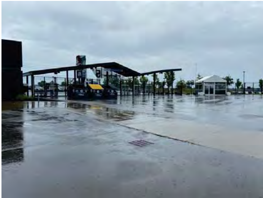
Photo 60 : Storm drain on exterior of Building One
