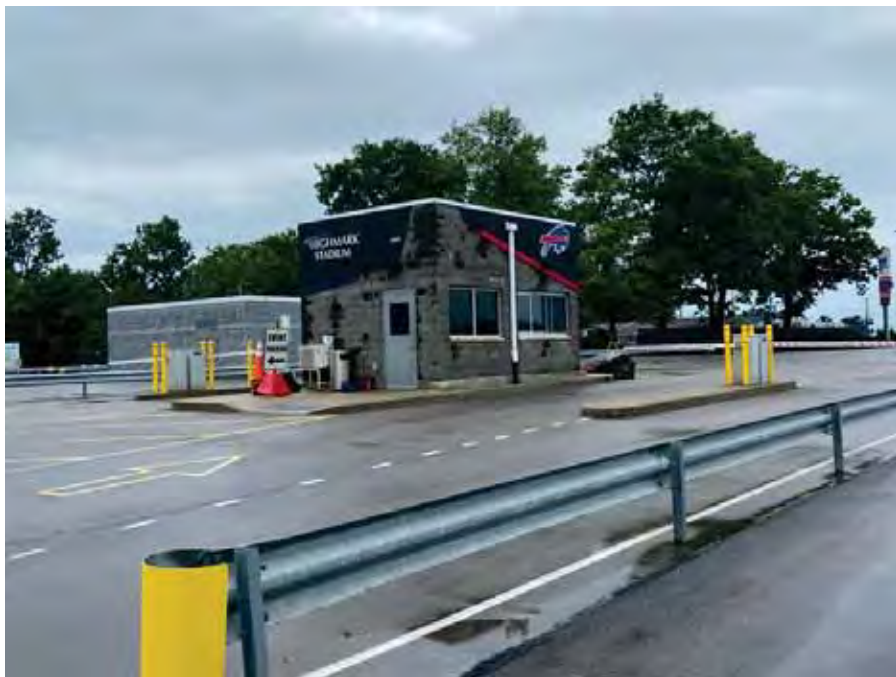
Photo 90 : Security Building on Area One
