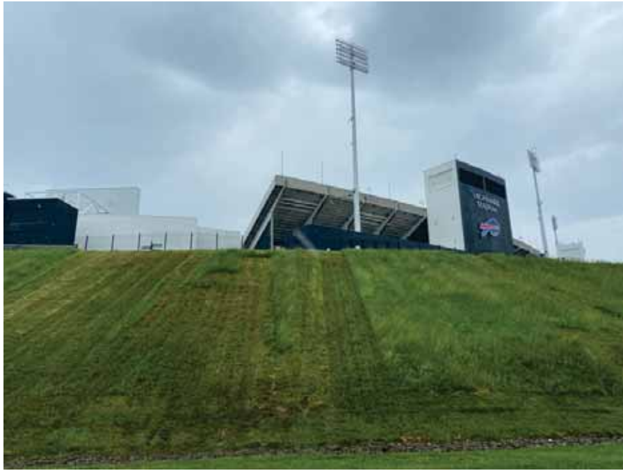
Photo 7 : Eastern exterior of Building One
