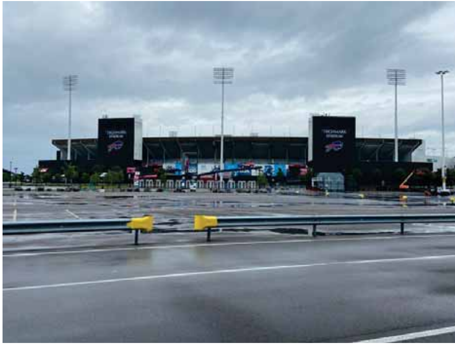
Photo 11 : Southern exterior of Building One
