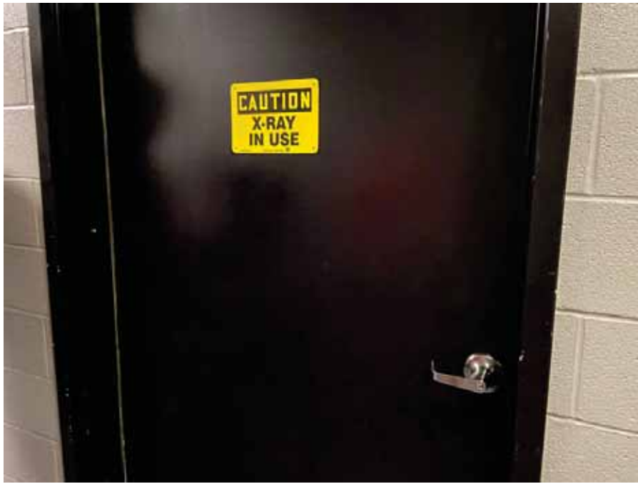
Photo 17 : X-Ray room within Building One
