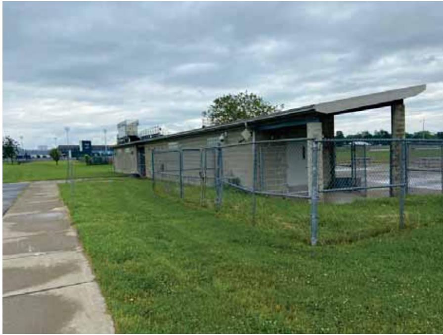
Photo 123 : Northern exterior of Building Nine
