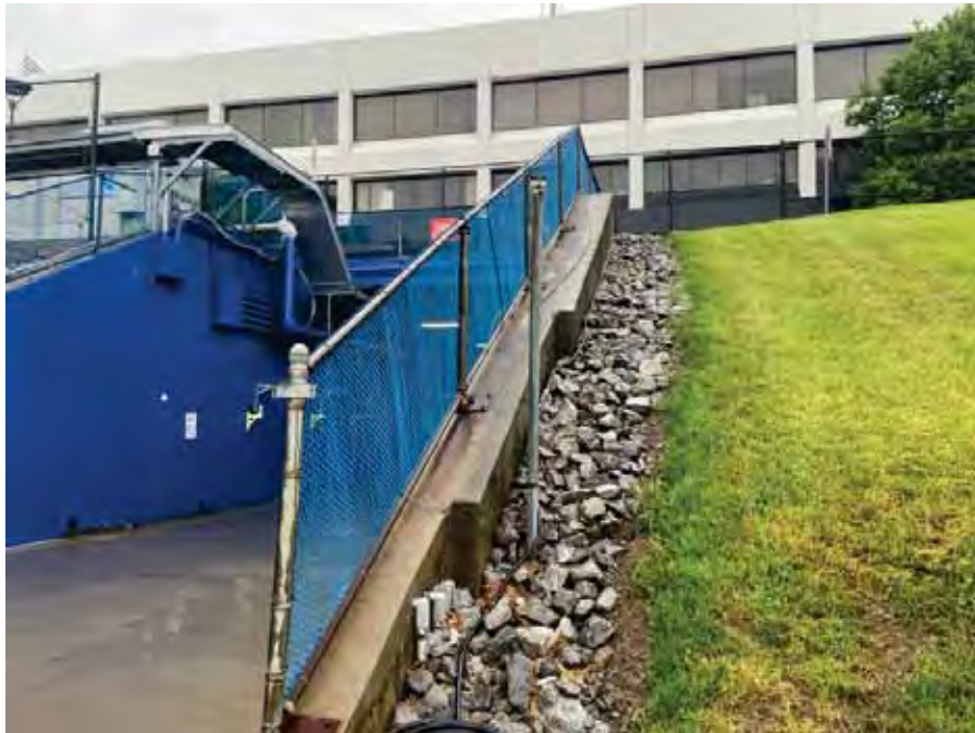
Photo 52 : Vent pipe next to tunnel
