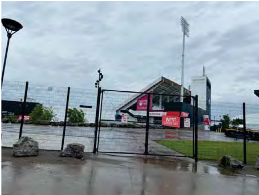
Photo 8 : Western exterior of Building One
