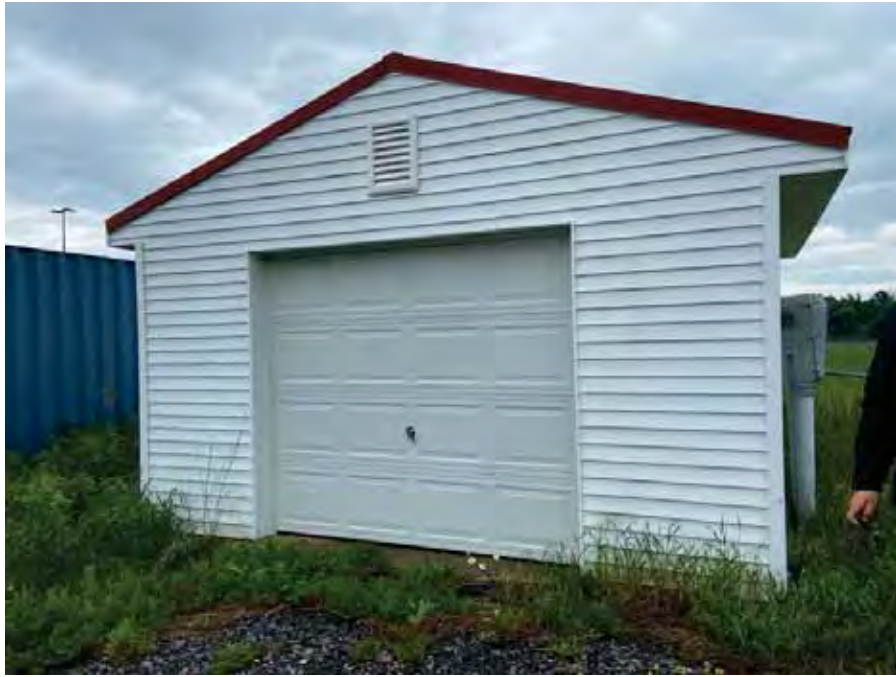
Photo 137 : Electrical building located on Area Two
