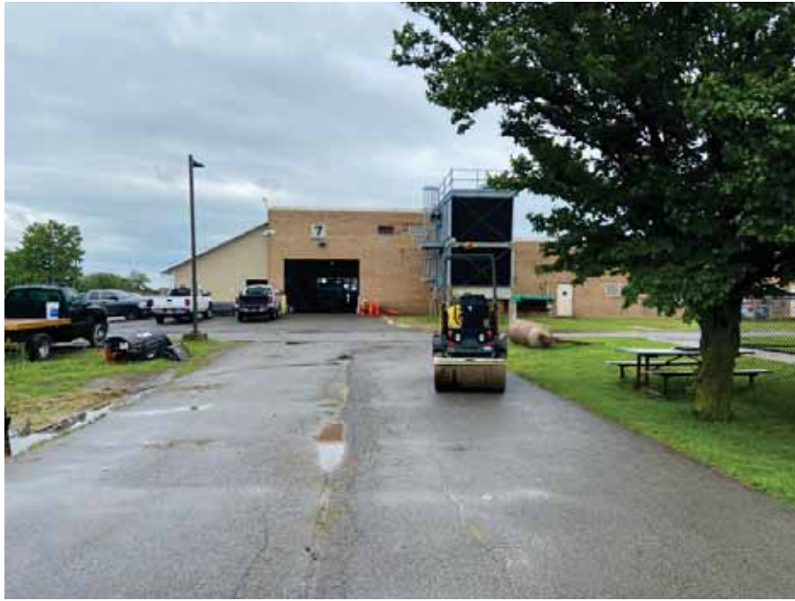
Photo 153 : Maintenance Building located West of Area Two
