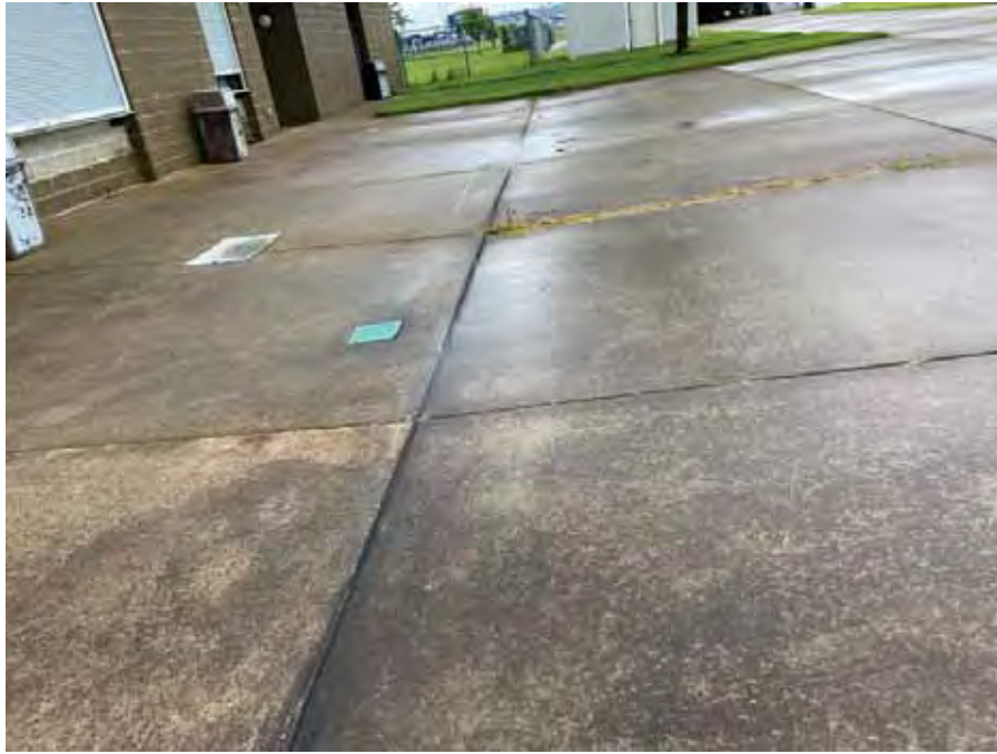
Photo 129 : Storm drains located south of Building Nine
