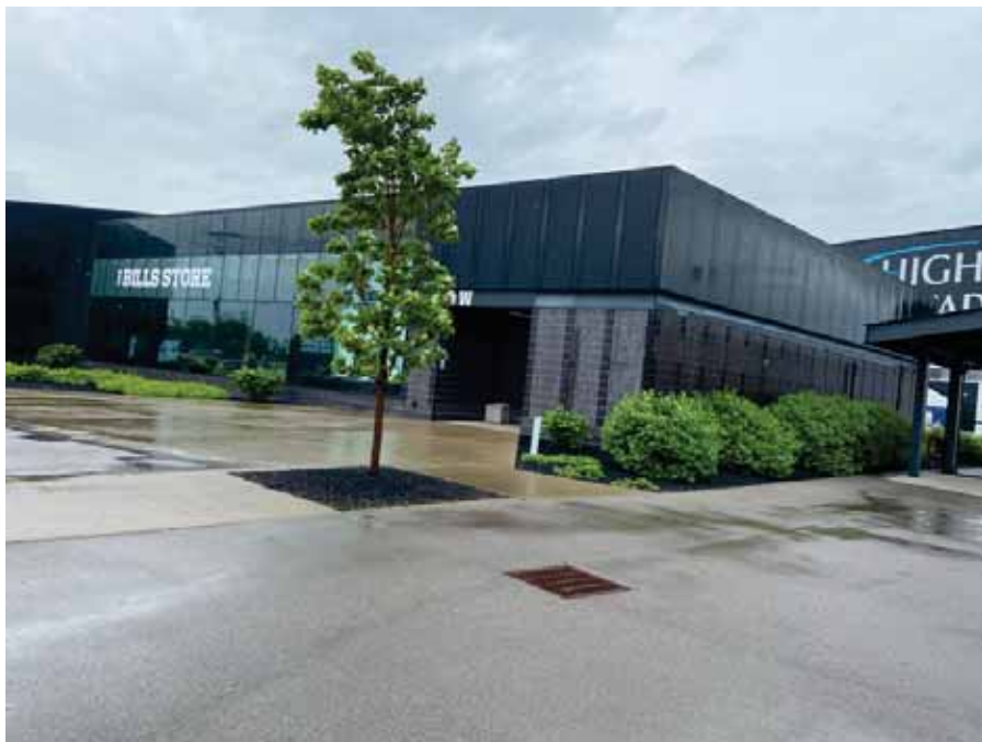
Photo 74 : Southern exterior of Building Three
