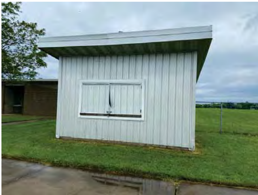
Photo 122 : Vendor shed located in Area Two
