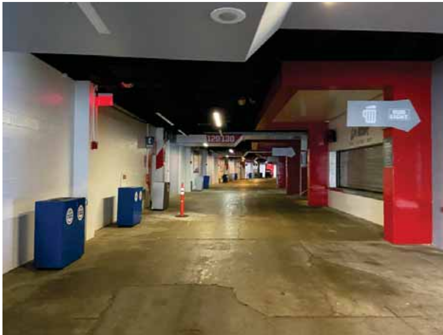
Photo 19 : Typical fan area within Building One
