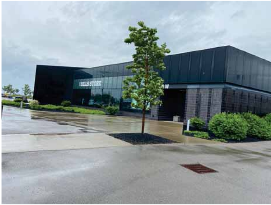
Photo 73 : Western exterior of Building Three
