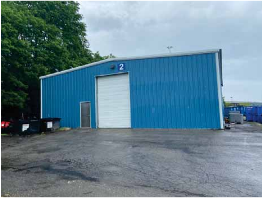
Photo 81 : Southern exterior of Building Four
