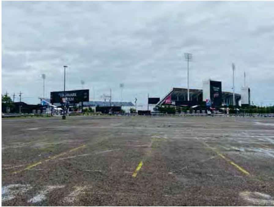
Photo 9 : Western exterior of Building One
