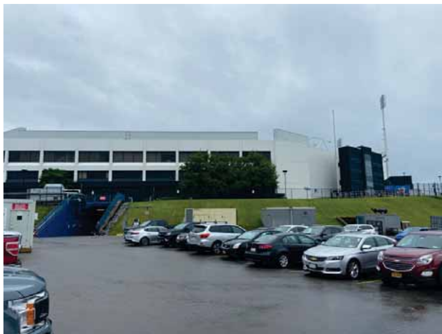
Photo 64 : Eastern exterior of Building Two
