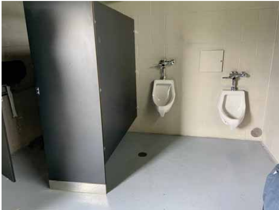
Photo 128 : Bathroom located in Building Nine
