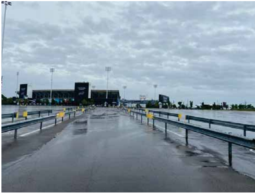
Photo 61 : Typical parking lot areas surrounding Building One
