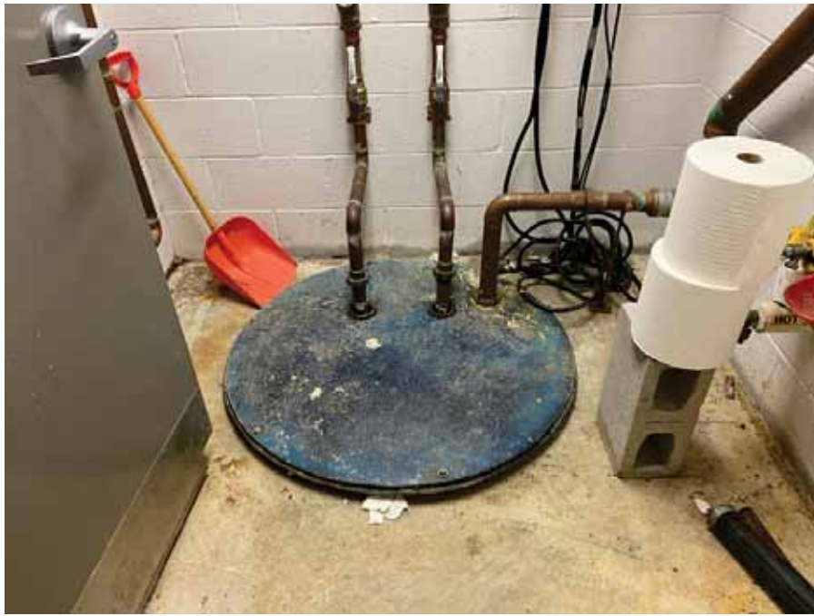
Photo 39 : Collection and pump located within Building Six
