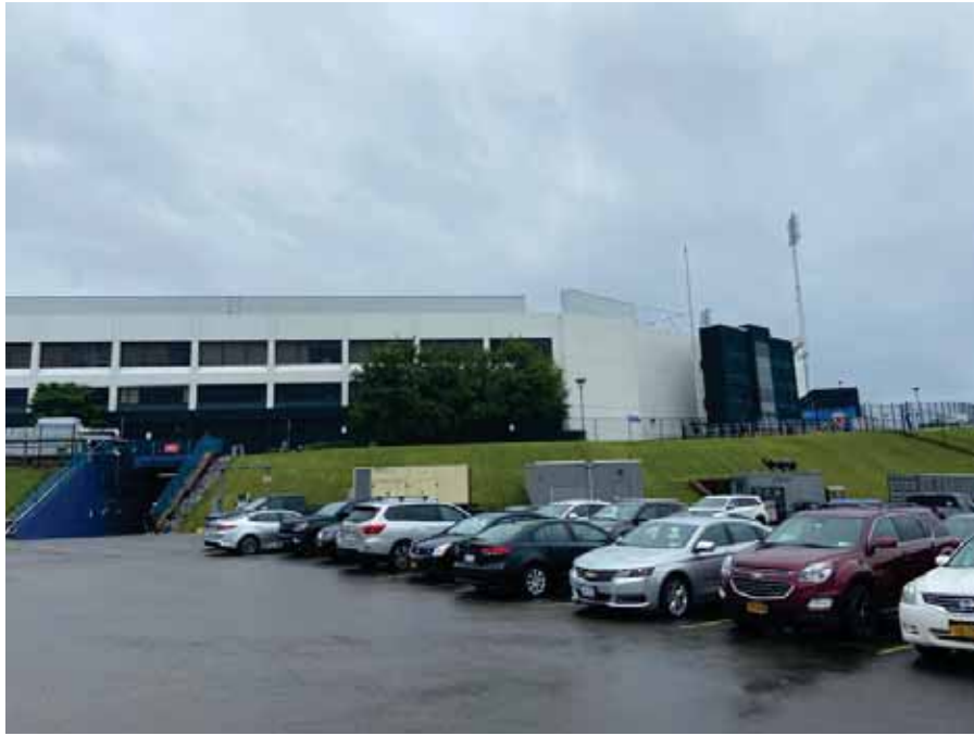
Photo 65 : Eastern exterior of Building Two
