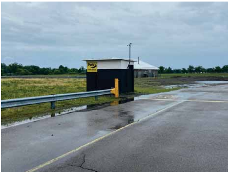
Photo 100 : Typical ticket boxes in Area One
