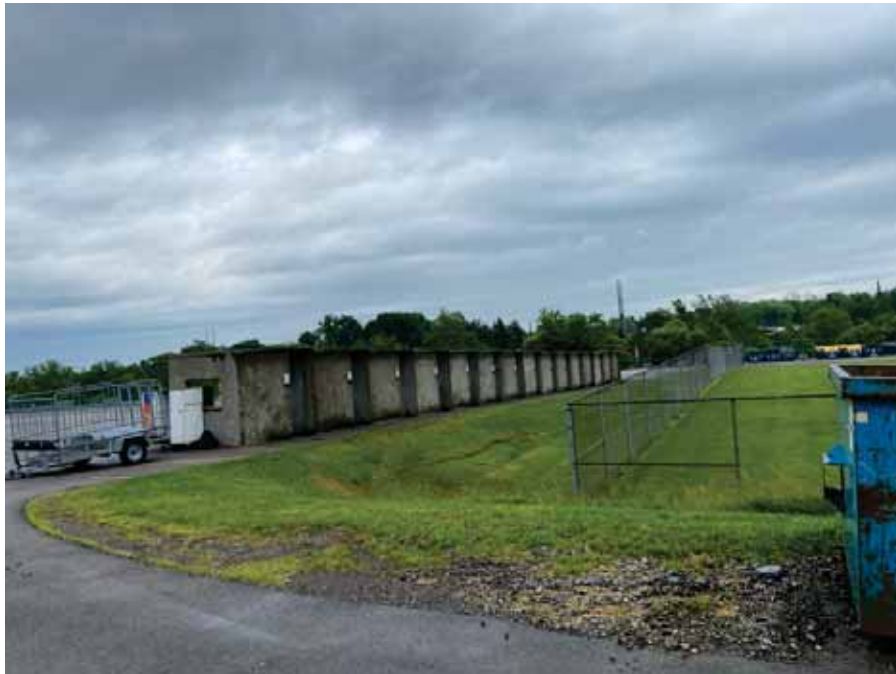
Photo 104 : Former vendor buildings in parking lot area north of Building One
