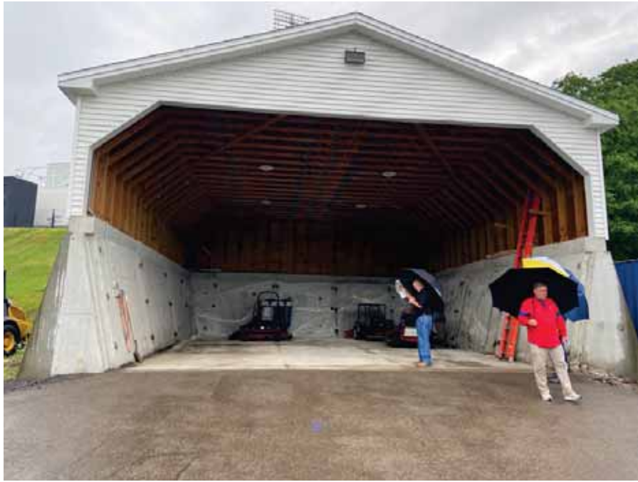
Photo 89 : Interior of Building Five
