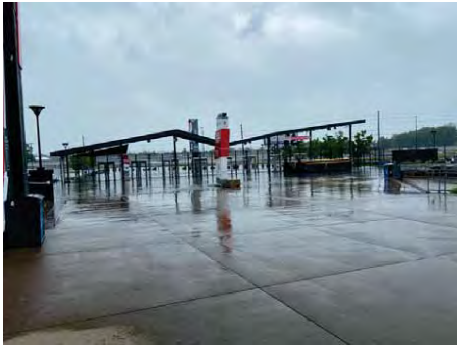
Photo 3 : Entrance area to stadium (Building One)
