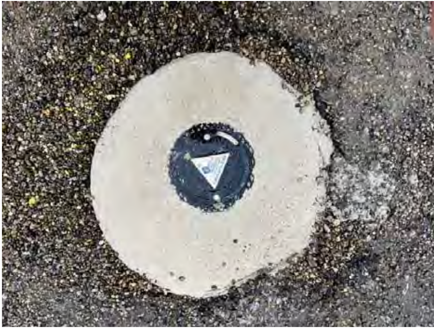
Photo 101 : Typical monitoring well in parking lot portion of Area One
