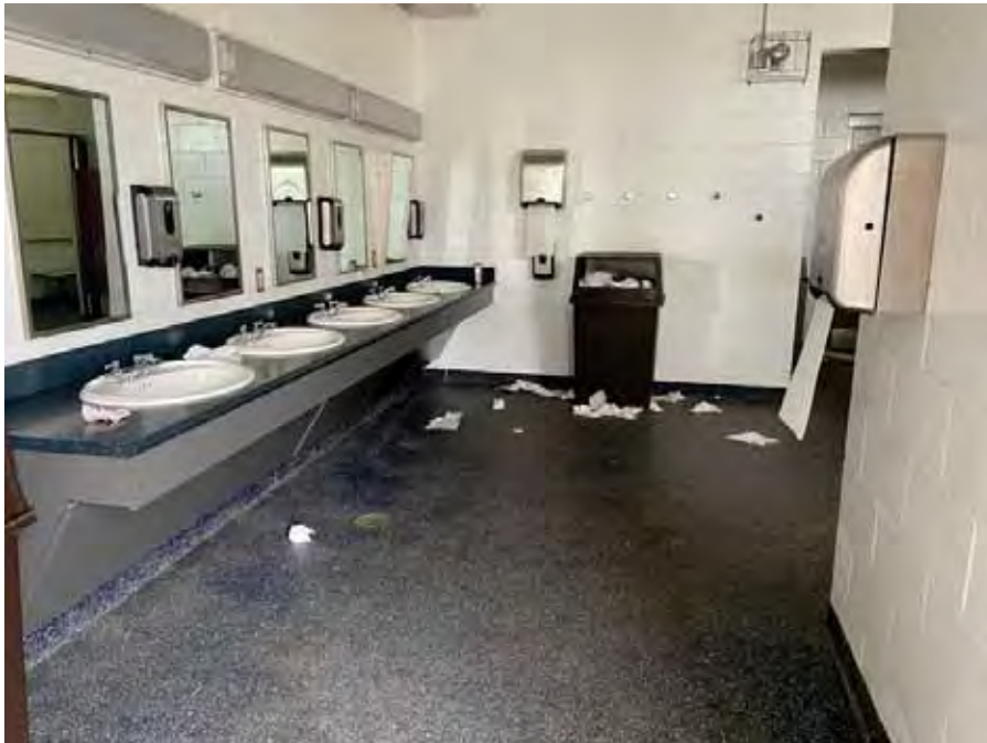
Photo 92 : Interior of Building Six
