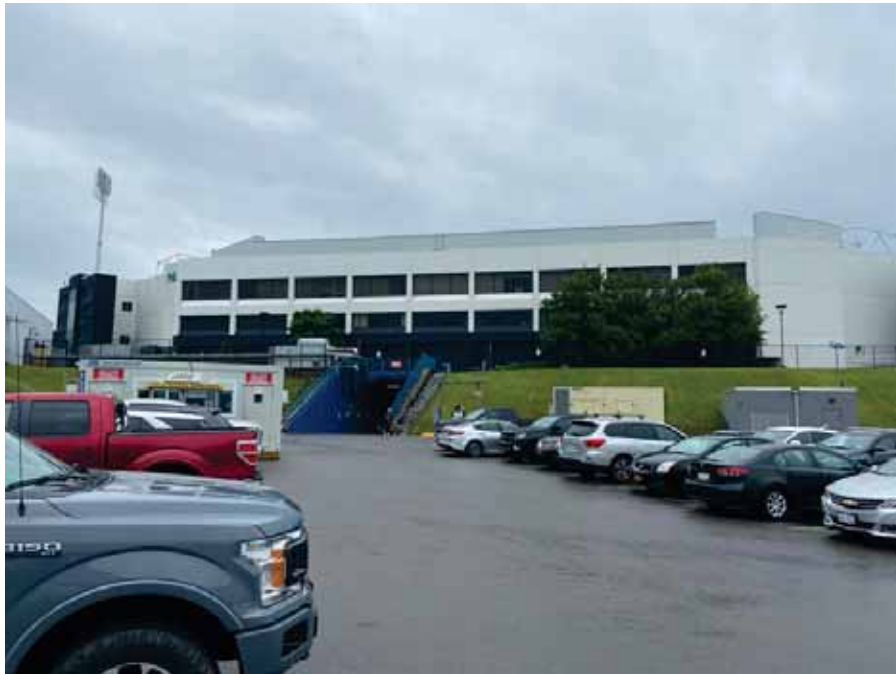
Photo 66 : Eastern exterior of Building Two
