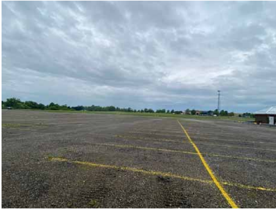
Photo 103 : Parking lot area across of Abbott Road located in Area One
