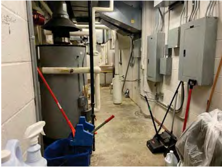
Photo 93 : Area within Building Six
