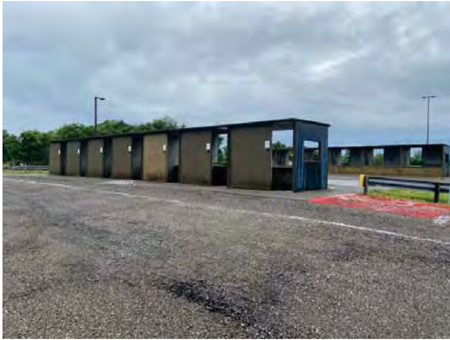
Photo 97 : Former vendor buildings in the parking lot area of Area One
