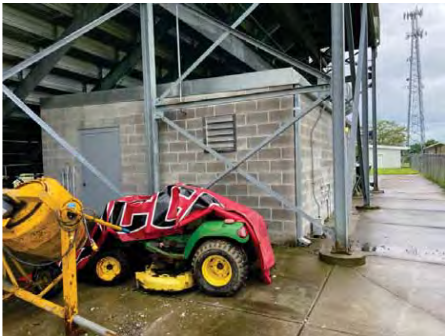
Photo 132 : Storage building underneath bleachers on Area Two
