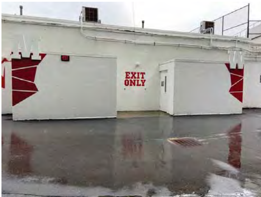
Photo 28 : Typical bathrooms and storm drain in Building One
