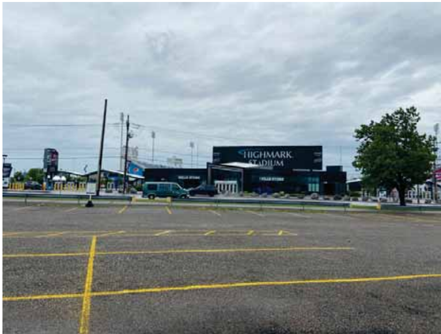
Photo 71 : Western exterior of Building Three
