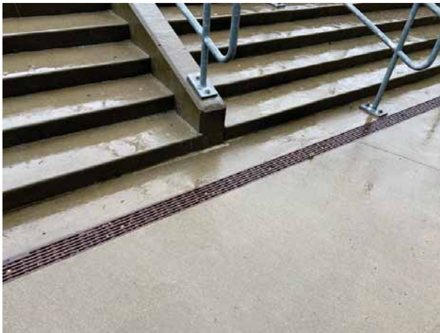
Photo 32 : Typical trench drain in Building One
