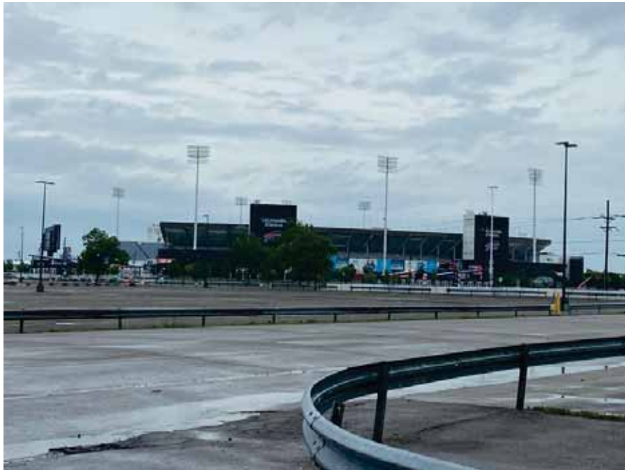
Photo 12 : Southwestern exterior of Building One
