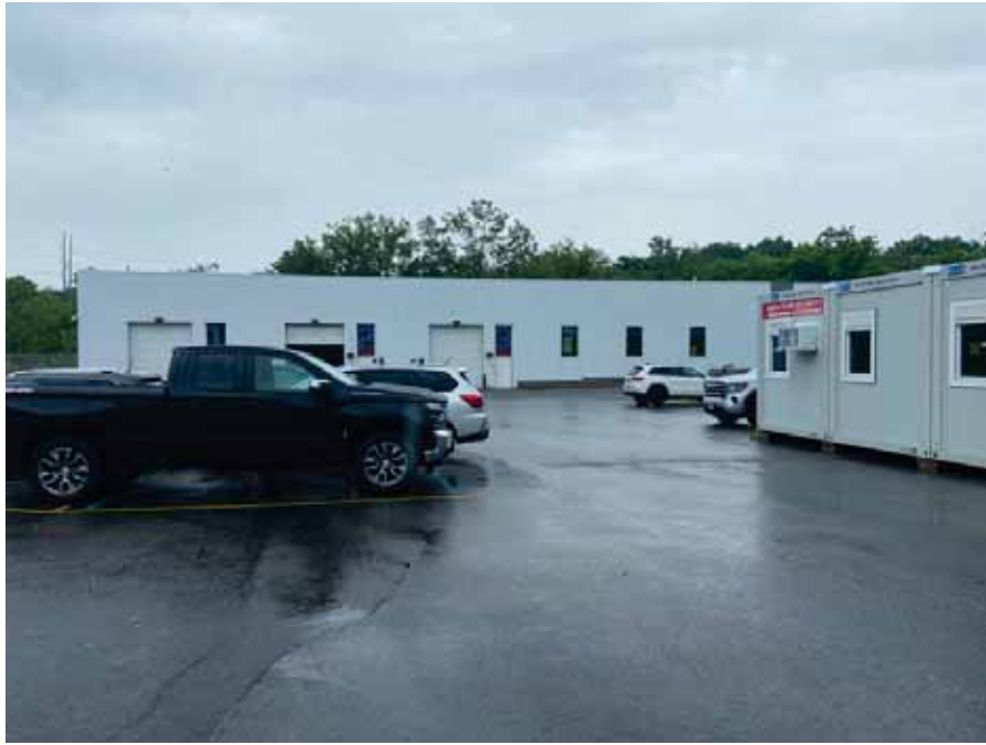
Photo 51 : Eastern Areas of Building One
