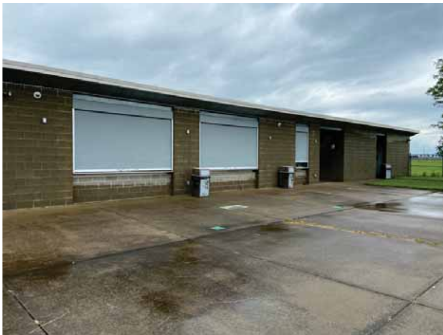
Photo 124 : Southern exterior of Building Nine
