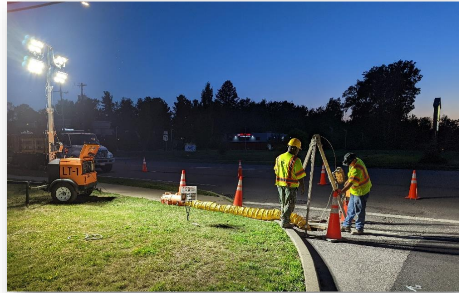
Sanitary sewer lining work in the Town of Clarence (ECSD No. 5)
