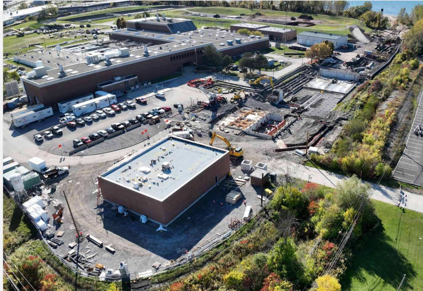
Phase 1 includes new electrical substation, effluent pumping station, chlorine contact tank, outfall repairs, and associated improvements (ECSD No. 3, Town of Hamburg)
