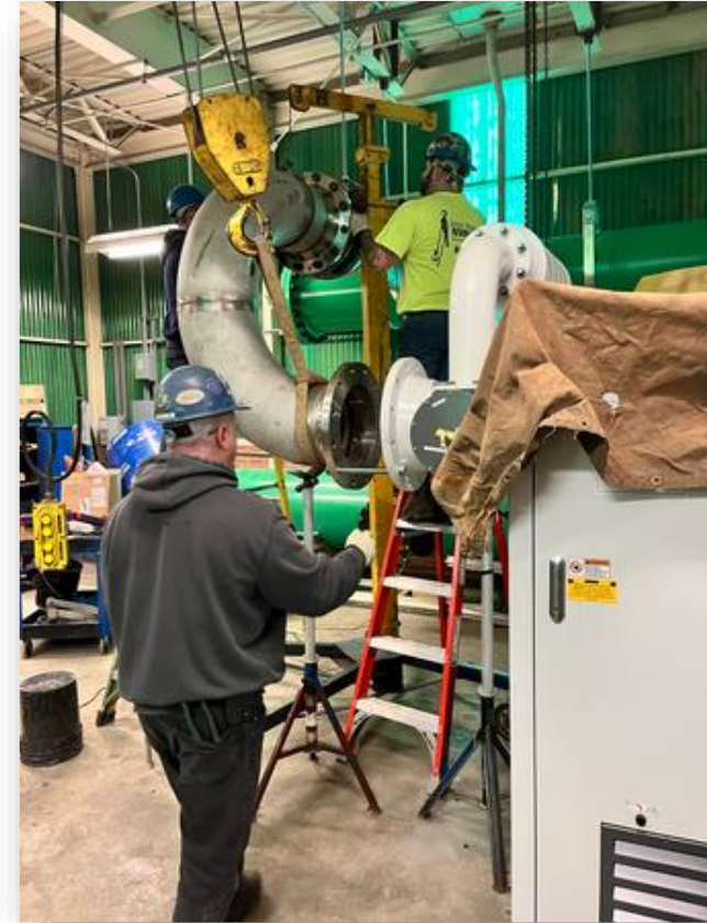
Blower replacement work at the Big Sister Creek WRRF (ECSD No. 2, Town of Evans)
