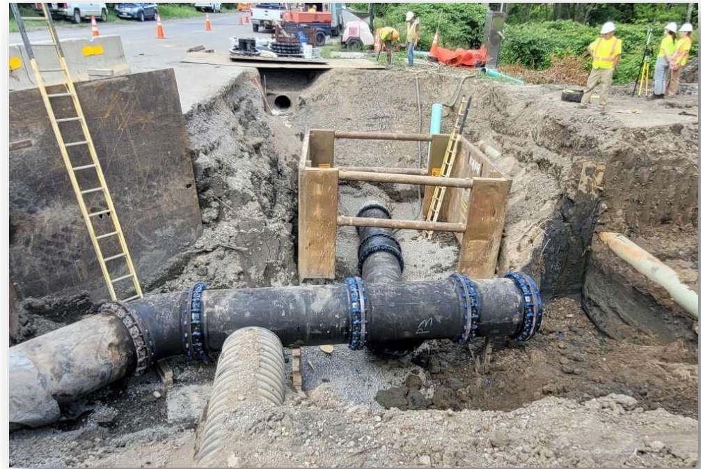
Force main replacement work in the Village of Depew (ECSD No. 4)
