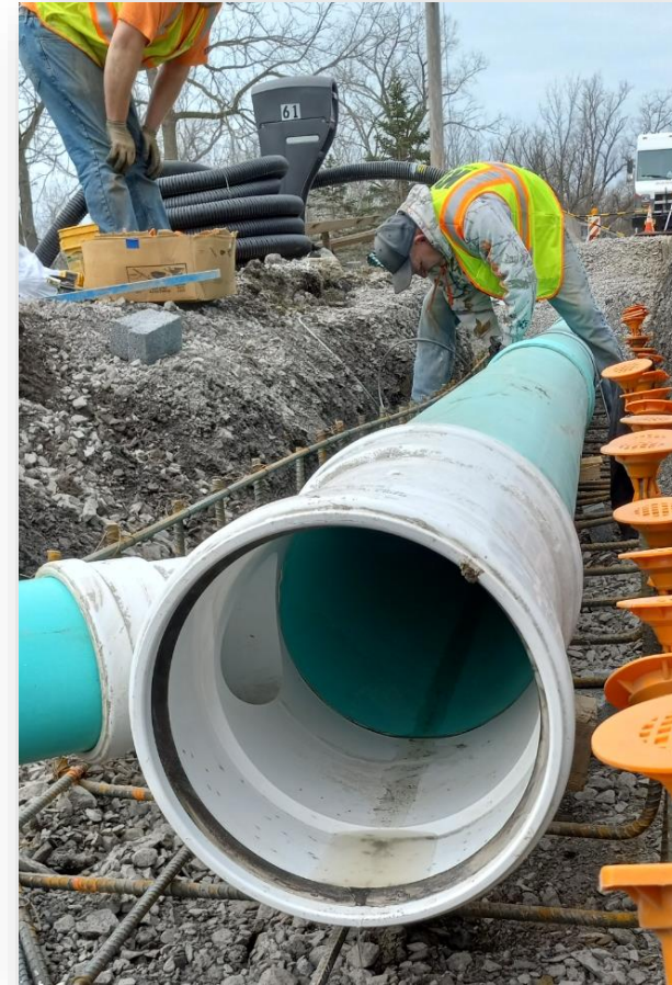
Sanitary sewer replacement work in the Town of Cheektowaga (ECSD No. 1)
