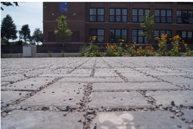
Permeable Pavers By: Mississippi Watershed Management Organization Source: Flickr
