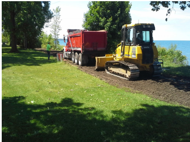
Point Gratiot Park, Paved Path - After removal—topsoiling
