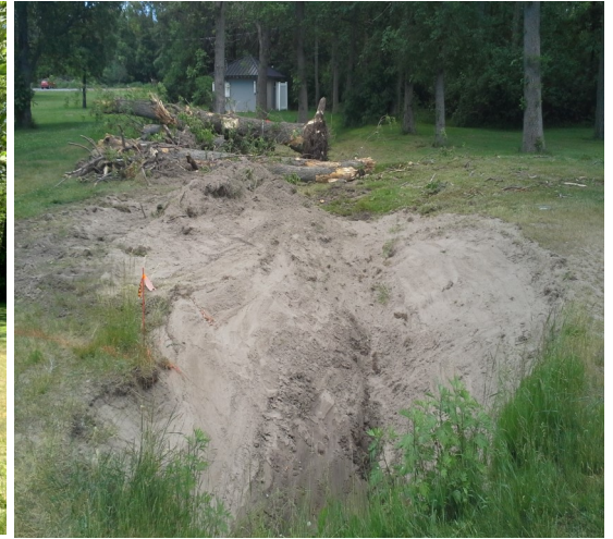
Park Drive Vegetated Swale/ Rain Garden—During construction
