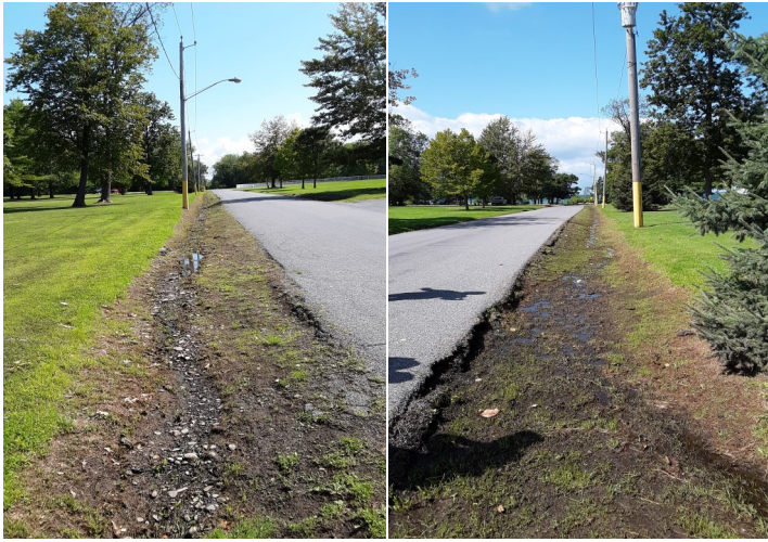
West Oak Street, Vegetated Swale — During construction, grading
