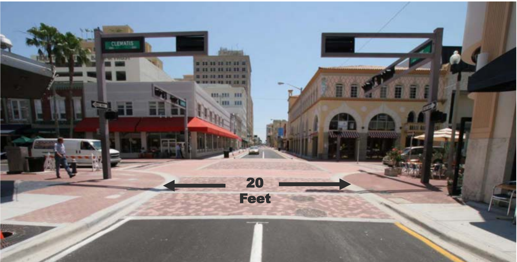
West Palm Beach's Olive Avenue is a Federal road. By taking its former 3-lane, 36 foot wide intersection down to two lanes, traffic moved slower and better. Why, pedestrian could cross in half of the time.
