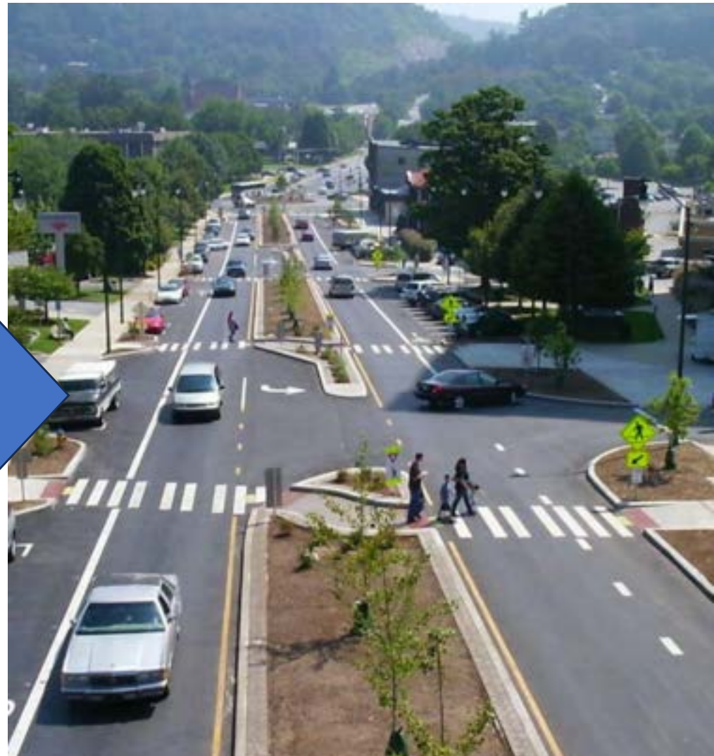
Asheville, NC had numerous serious crashes, especially to pedestrians. The solution required narrowing this street, which was only made possible by building a roundabout to keep traffic moving.
