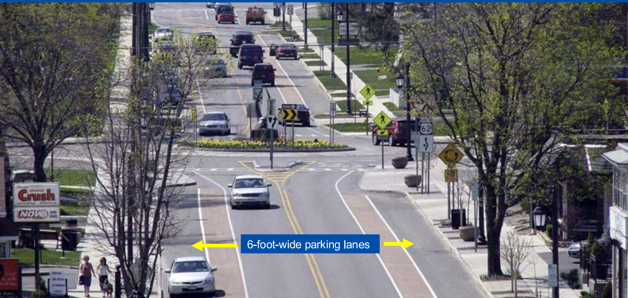
Hamburg, New York, narrowed travel lanes on US Route 62 to 10 feet and saw injury crashes decline by 60 percent and serious injuries fall by 90 percent on the corridor. Photo by Dan Burden.
