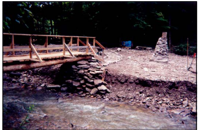
Wood products and limestone from Erie County Forest were used to construct this bridge to an island deep in the woods on Lot 2. Fifteen bridges were recently built to reconnect many miles of hiking trails.
