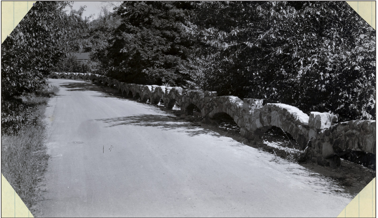
Stone work construction/road guardrails built by the WPA at Chestnut Ridge Park.
