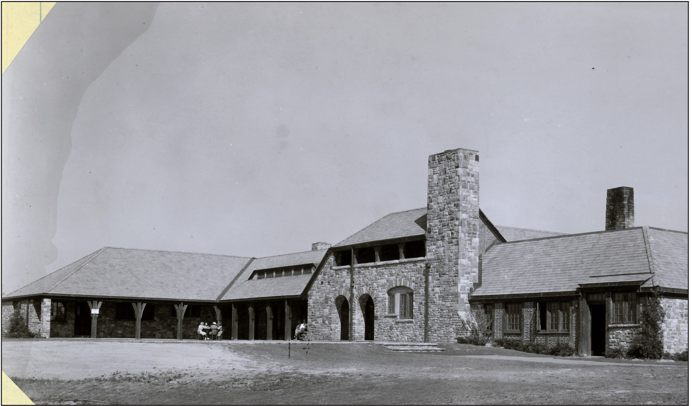
The Chestnut Ridge Park Casino was built in 1938 as a WPA project. The original casino was built in 1925, but was destroyed by fire.
