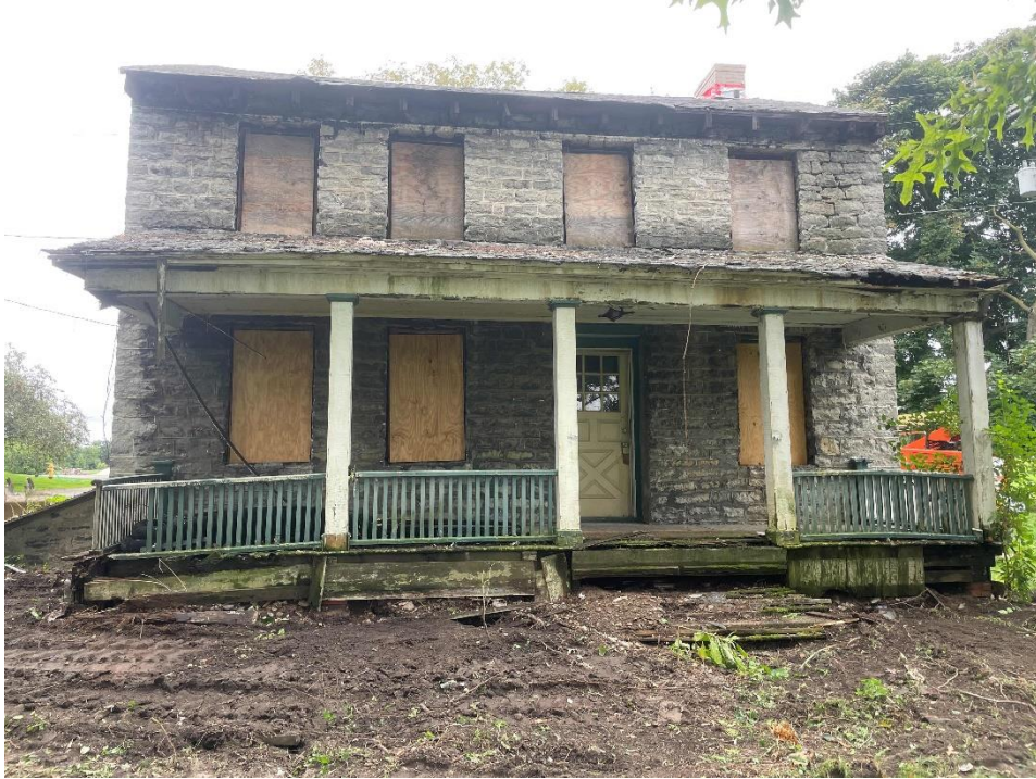
Schenck House (2022) at start of construction with non-original porch still intact.
