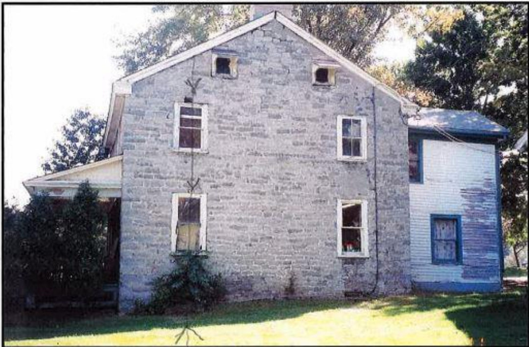
PHOTO 2. View of Western Elevation Showing Wood Frame Addition.
