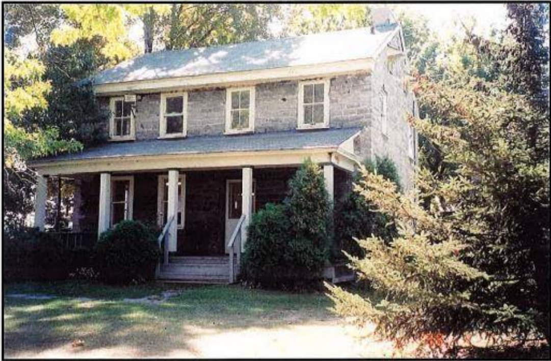
PHOTO 1. View of Northern Elevation.
