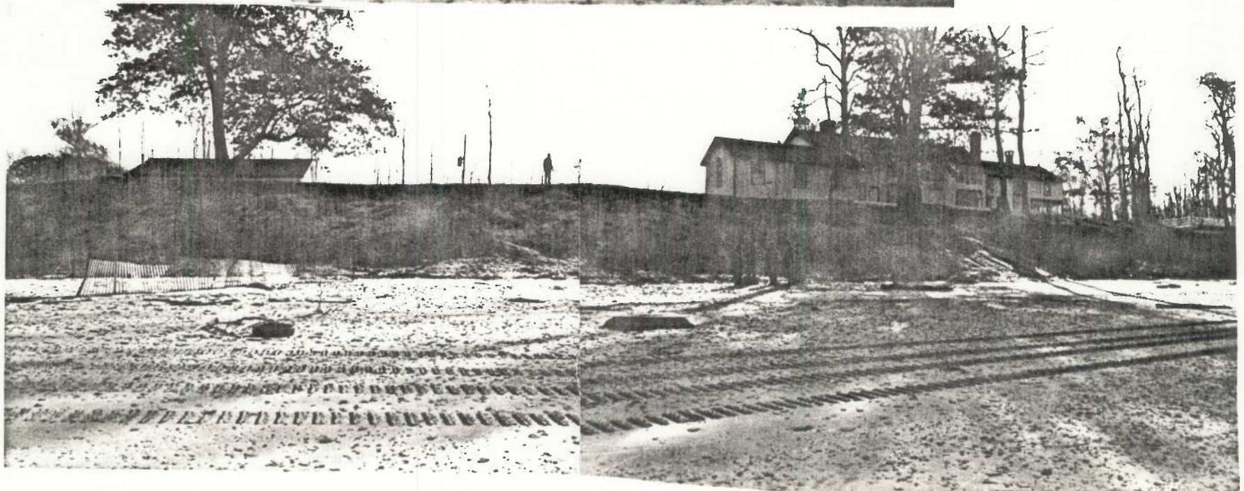
Wendt Beach Park - Before Construction Photos
