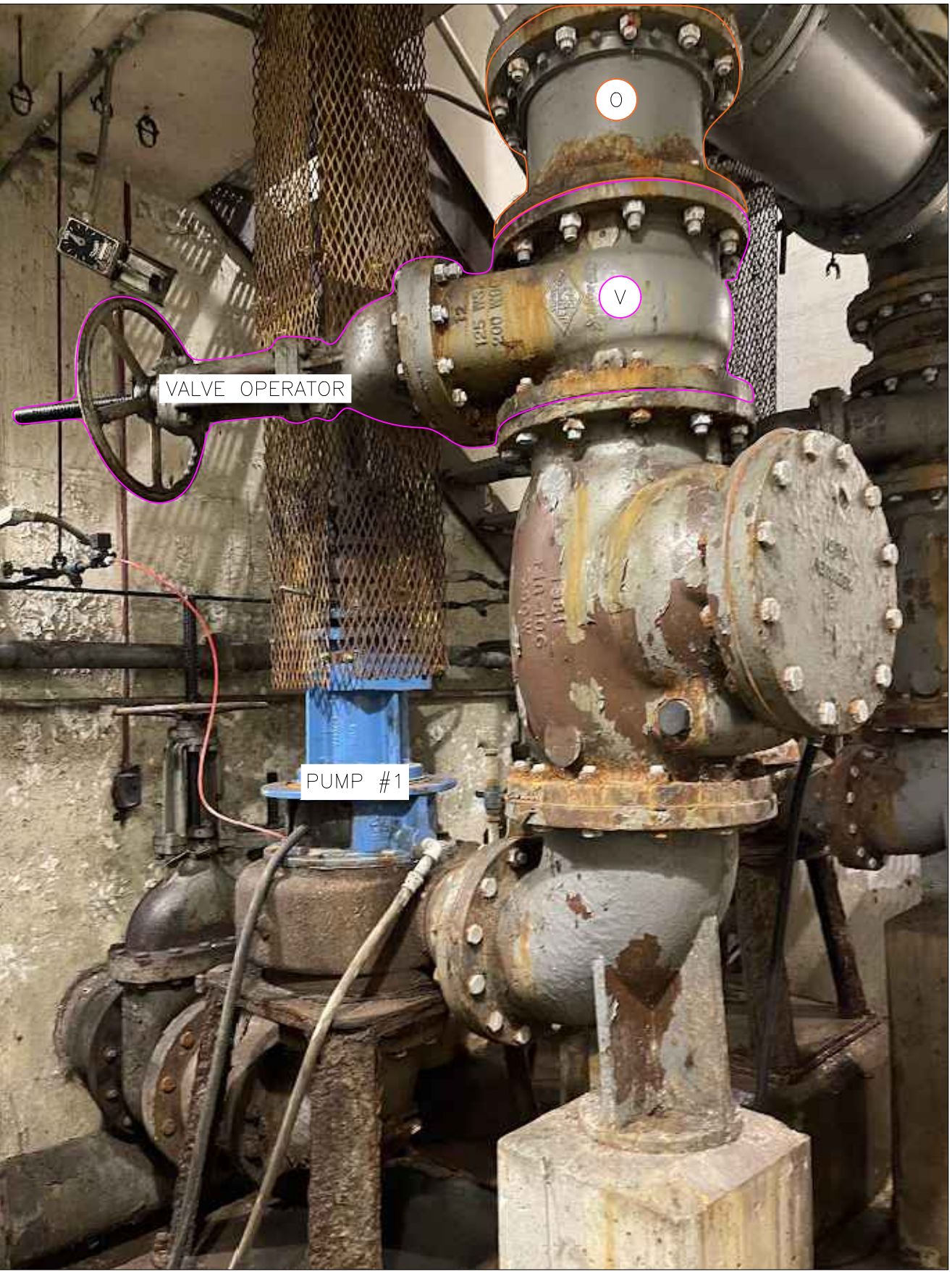
EXISTING PUMP NO. 1 VALVE DIRECTION (SEE NOTE 4)
